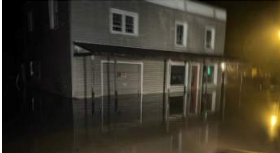
Figure 624: Flooding in Bandy, VA in July 2022 40
