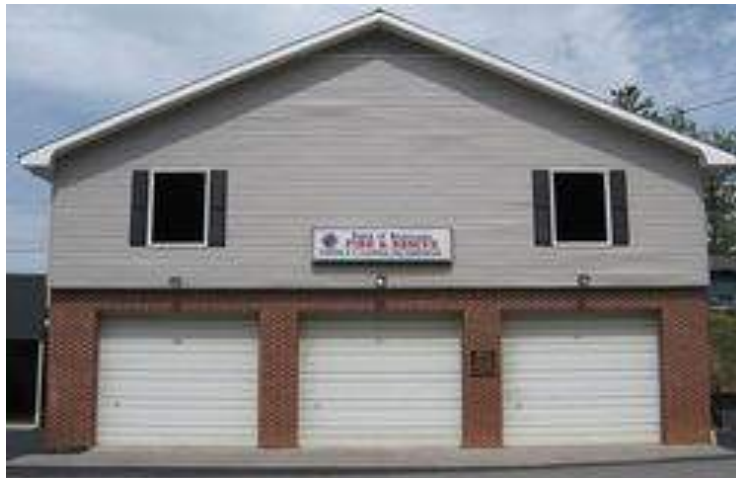
Figure 75: Richlands Fire-Rescue Station 3
