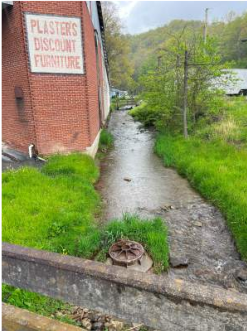
Figure 726: Plasters Discount Furniture alongside Mill Creek during regular conditions
