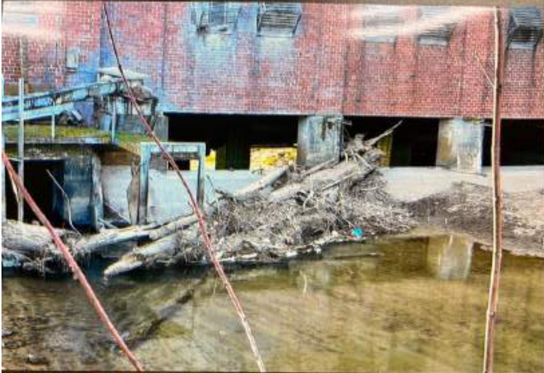
Figure 642: Debris Gathered on Upstream Side of Abandoned Mill Building in North Tazewell
