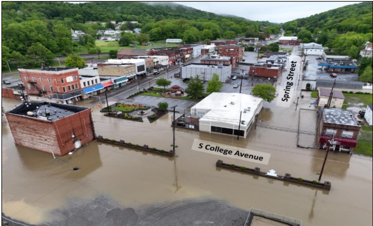
Figure 3: Flooding in Bluefield, Virginia- May 29, 2023
