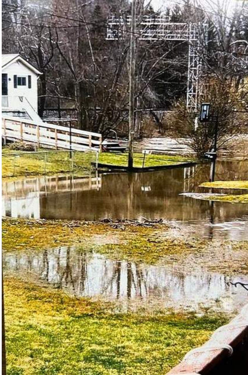
Figure 643: Floodwaters on the East End of Blacksburg Street
