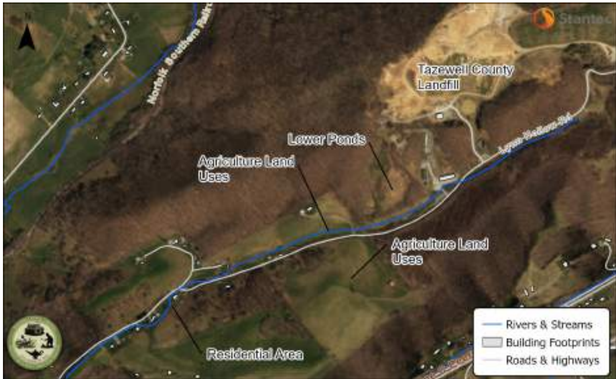
Figure 723: Lynn Hollow Road Area
