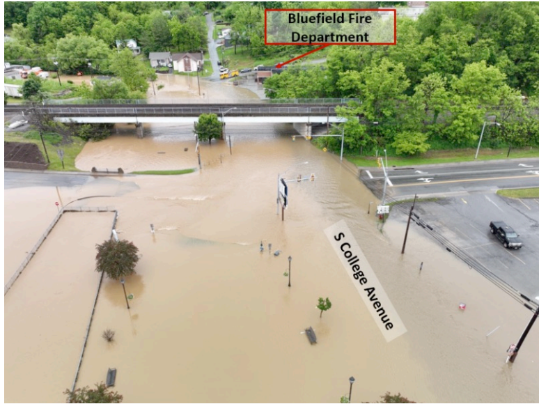
Figure 8: Flooding Blocking Access to the Bluefield Fire Department - May 29, 2023.
