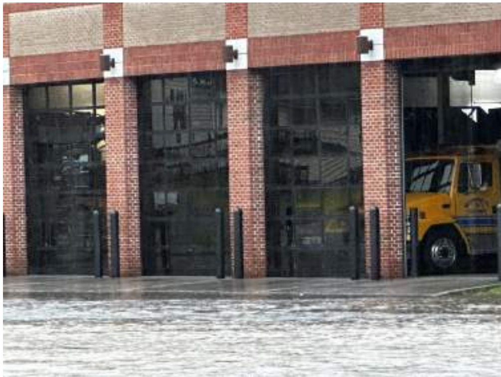
Figure 714: Flooding outside of the Bluefield Fire Department- May 29, 2023
