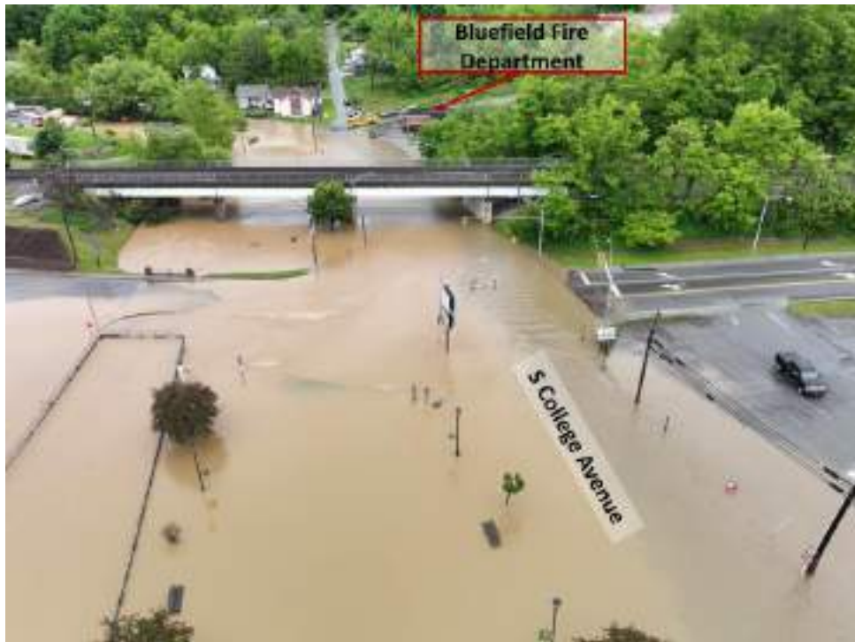
Figure 713: Flooding blocking access to the Bluefield Fire Department- May 29, 2023
