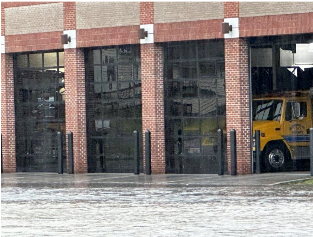
Figure 9: Flooding outside of the Bluefield Fire Department - May 29, 2023.
