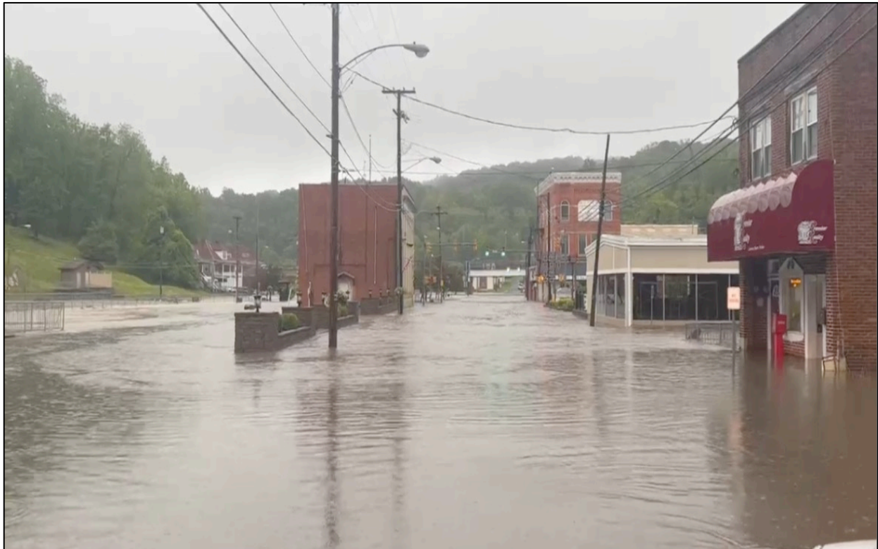
Figure 2: Flooding in Bluefield, Virginia- May 29, 2023
