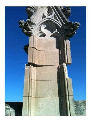
Figure 26: Earthquake Damage to Washington National Cathedral in Washington, D.C. After the 2011 Earthquake<sup>77</sup>
