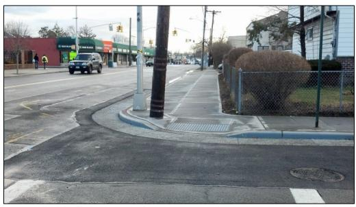
Figure 6. Permeable Concrete Gutter Installation
