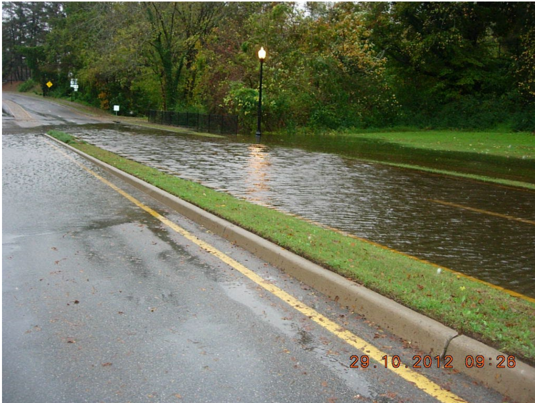
Flooding of E. Constance Road (U.S. 58 Business) during Hurricane Sandy in October 2012. Photo is looking eastbound towards Chesapeake.
