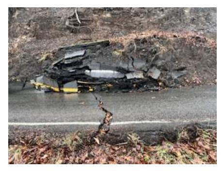
Figure 647: Damage from Landslide Event on Route 91
