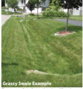
Grassy swales along streets without sidewalks could address street flooding by providing holding space for stormwater during rain events -- swales are designed to drain after rain event to avoid standing water. Swales can also be designed for ease of maintenance and to minimize trash collection.
