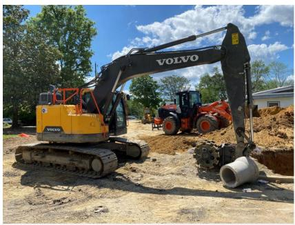
© James River Association. Construction equipment will be a common sight along Brunswick Street as crews install two sections of reinforced concrete pipe and a filter station to reduce problems with stormwater runoff.
