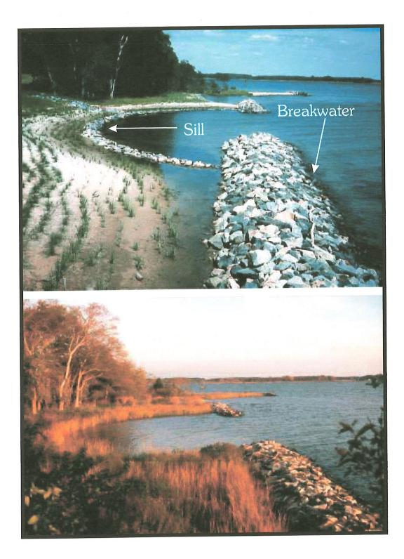
Figure 5. Stone sill connecting breakwaters with sand fill and marsh implantation on Choptank River, Talbot County, Maryland just after construction and 5 years post-construction (Hardaway and Byrne, 1999).
