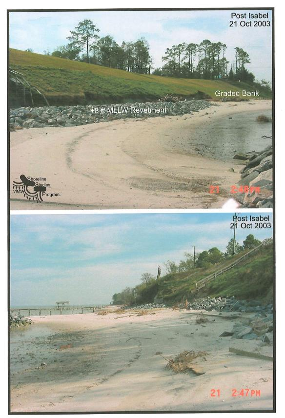
Figure 35. Impacts at the downriver end of Van Dyke where the shore is protected by a revetment.
