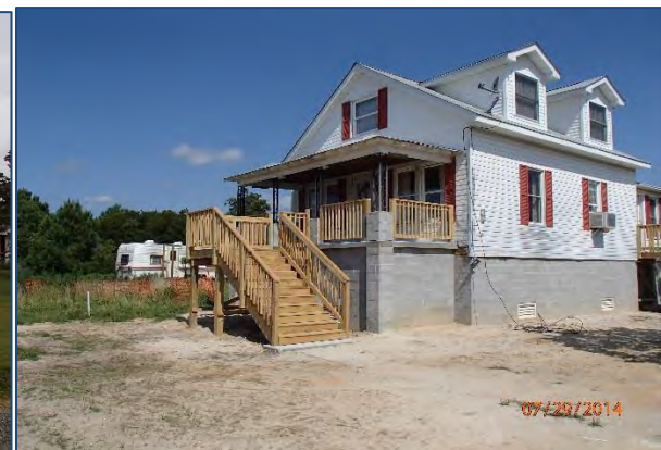
Figure 80: House in Hayes, Gloucester County - AFTER elevation.
