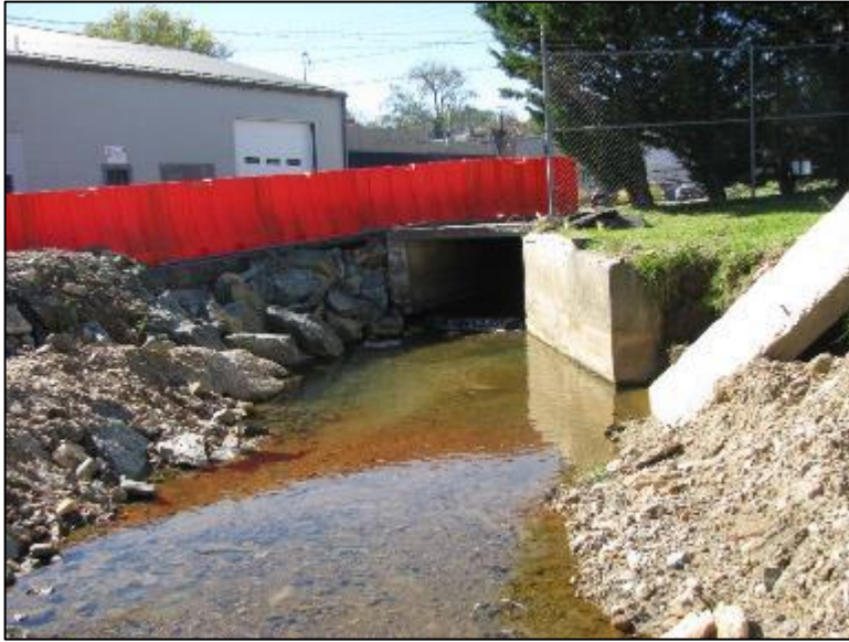
Box Culvert Outlet at Bartlett Street
