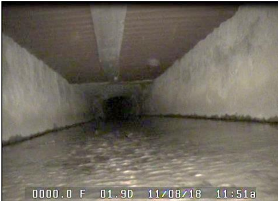
Internal View of Box Culvert Near Depot Street
