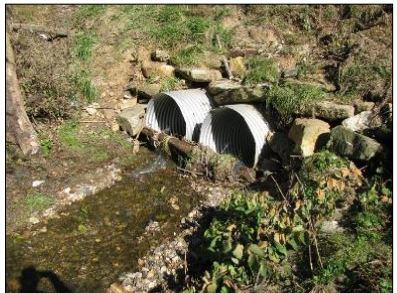
Inlet End of 42" Pipes at Playground
