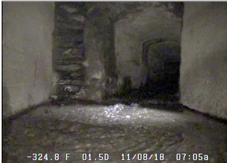
Box Culvert Transition at South Main Street
