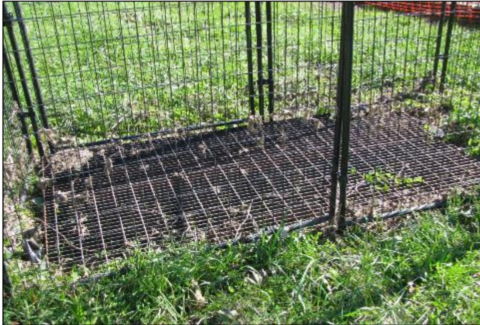
Drop Inlet Located in Galax Elementary Playground
