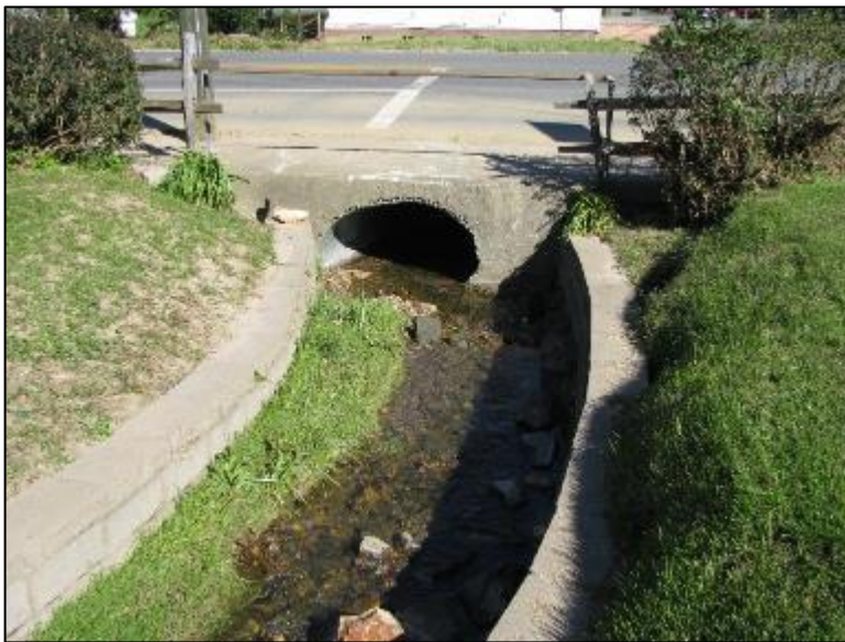
Inlet End of Pipe at McArthur & Swanson
