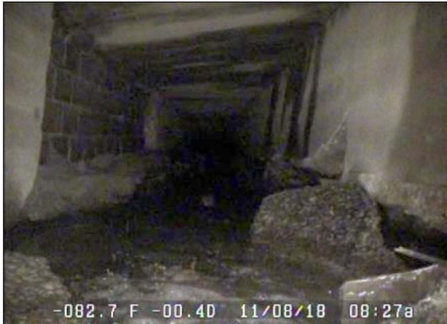
Inlet End of Box Culvert at Academy Street
