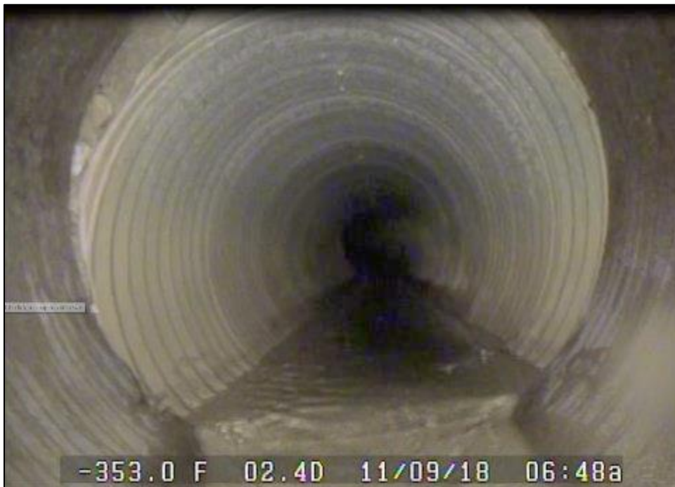
Transition from 24" HDPE to 24" CMP with Joint Offsets
