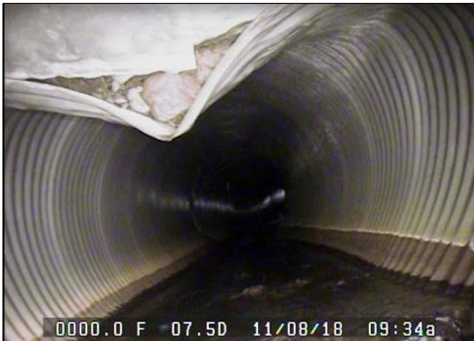
48" CMP Pipe Into Structure A12 at Swanson Street
