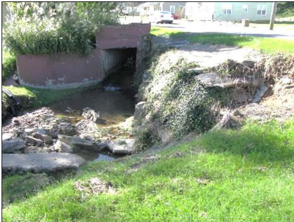
Discharge Outlet of Box Culvert at Swanson Street
