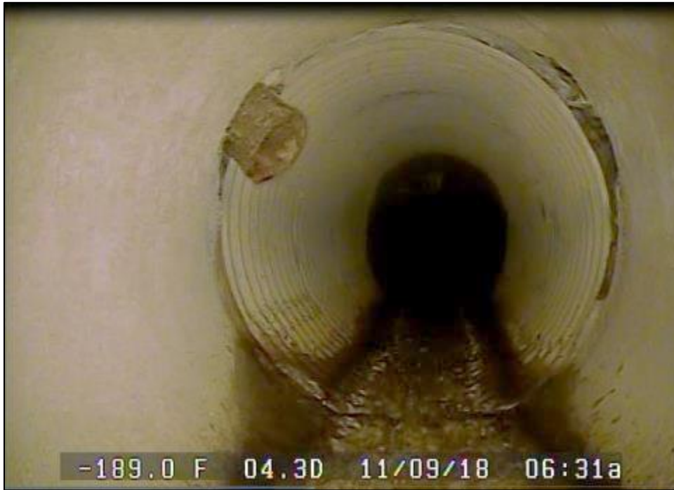
Transition from 24" RCP to 24" CMP Near Back of Oldtown Market Building
