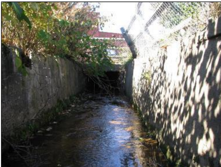
Outlet of Box Culvert Below Guynn Furniture
