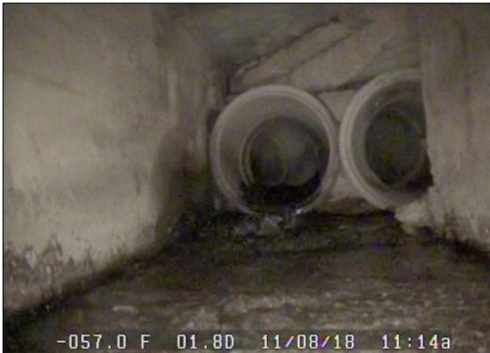
Transition from Box Culvert to 36" Pipe Beneath Swanson Street
