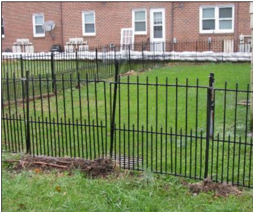
Sandbags at Madison Street Apartments
