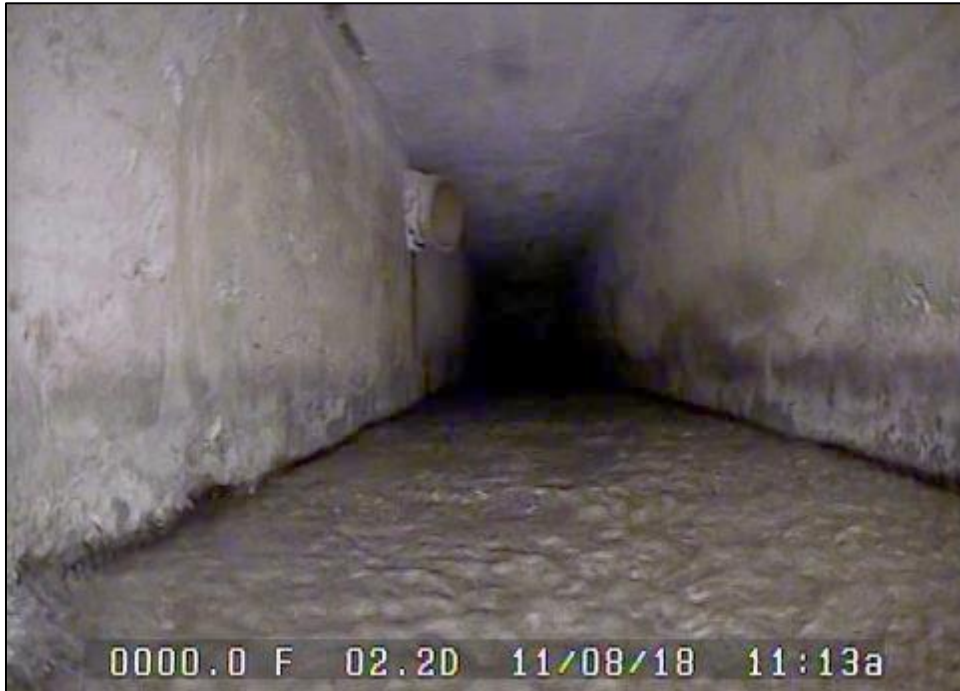
Interior of Box Culvert Beneath Swanson Street
