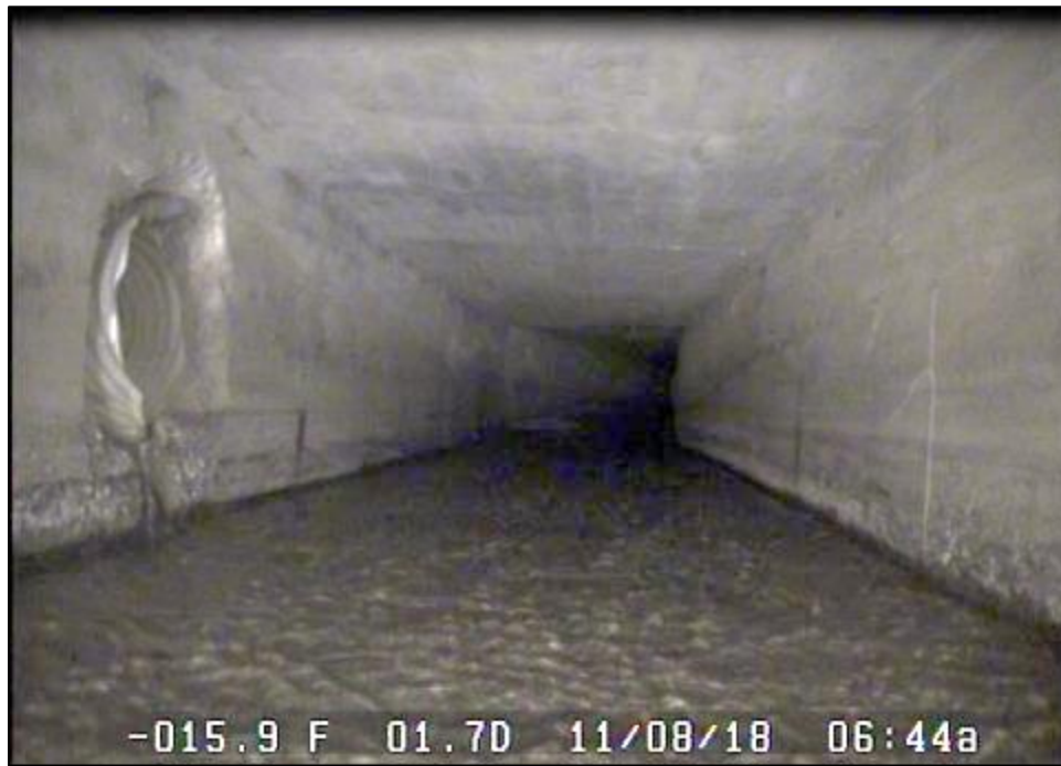
6' x 3.7' Box Culvert Under Bartlett Street
