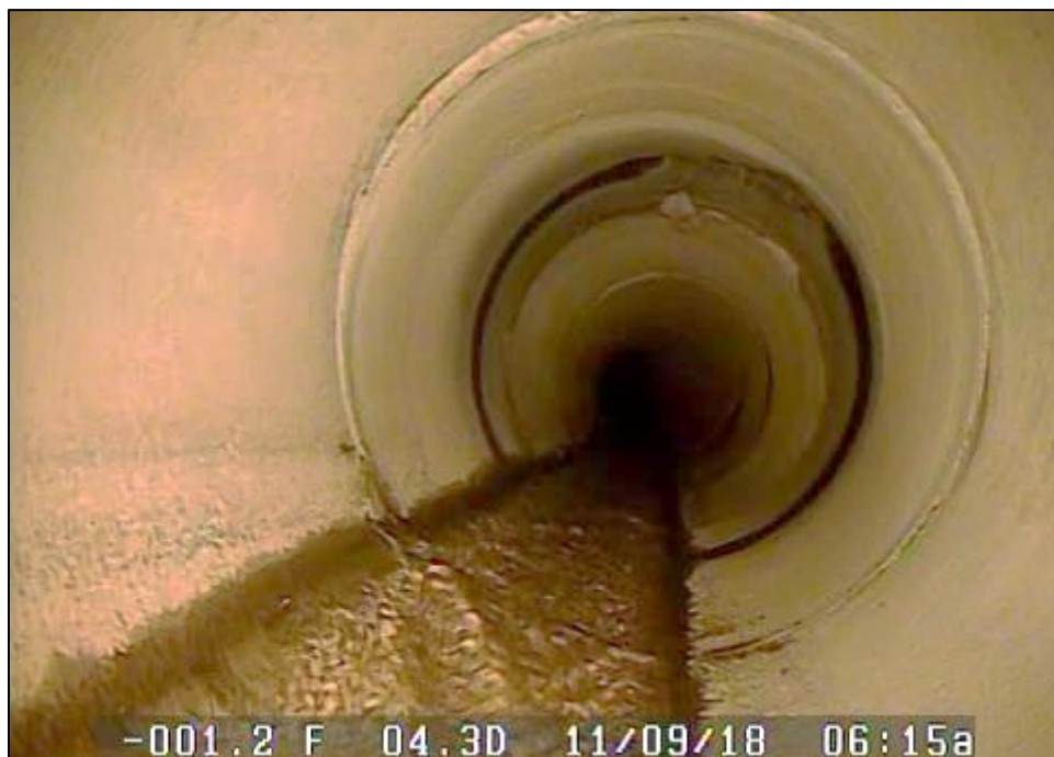
24" RCP Located Beneath Oldtown Market Parking Lot
