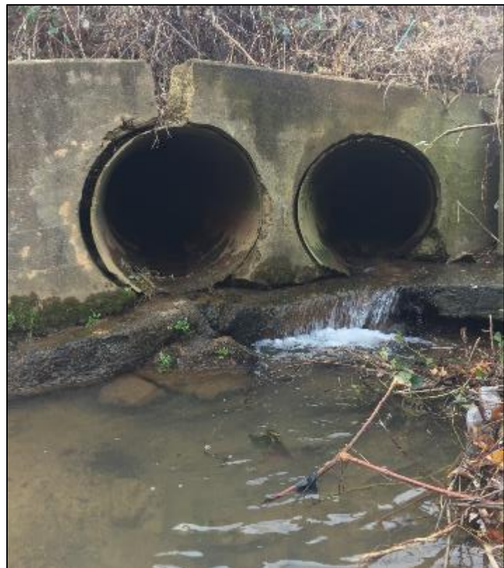
Outlet of Pipes Discharging to Chestnut Creek
