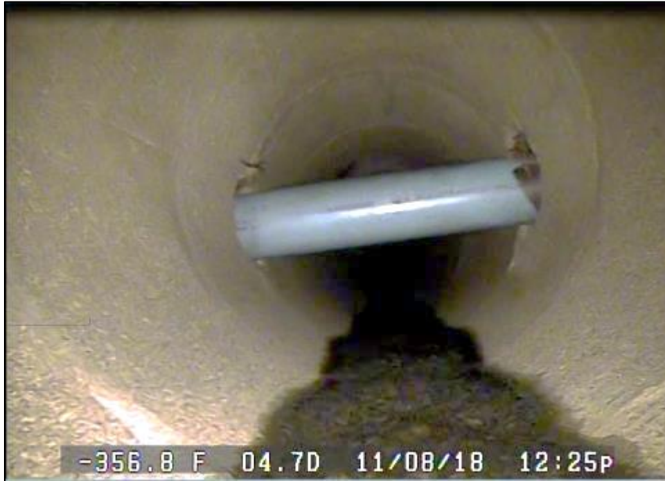
8" Water Line Installed Through 36" RCP at Carroll Street
