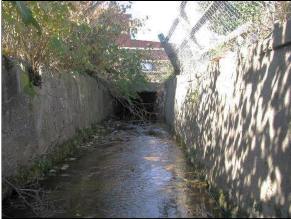
Outlet End of 6.33' x 3' Box Culvert Near Depot/Oldtown Streets
