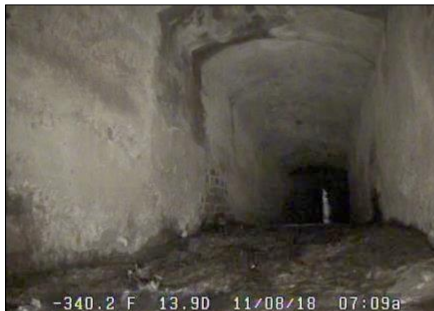
Smaller Box Culvert Section Upstream of South Main Street
