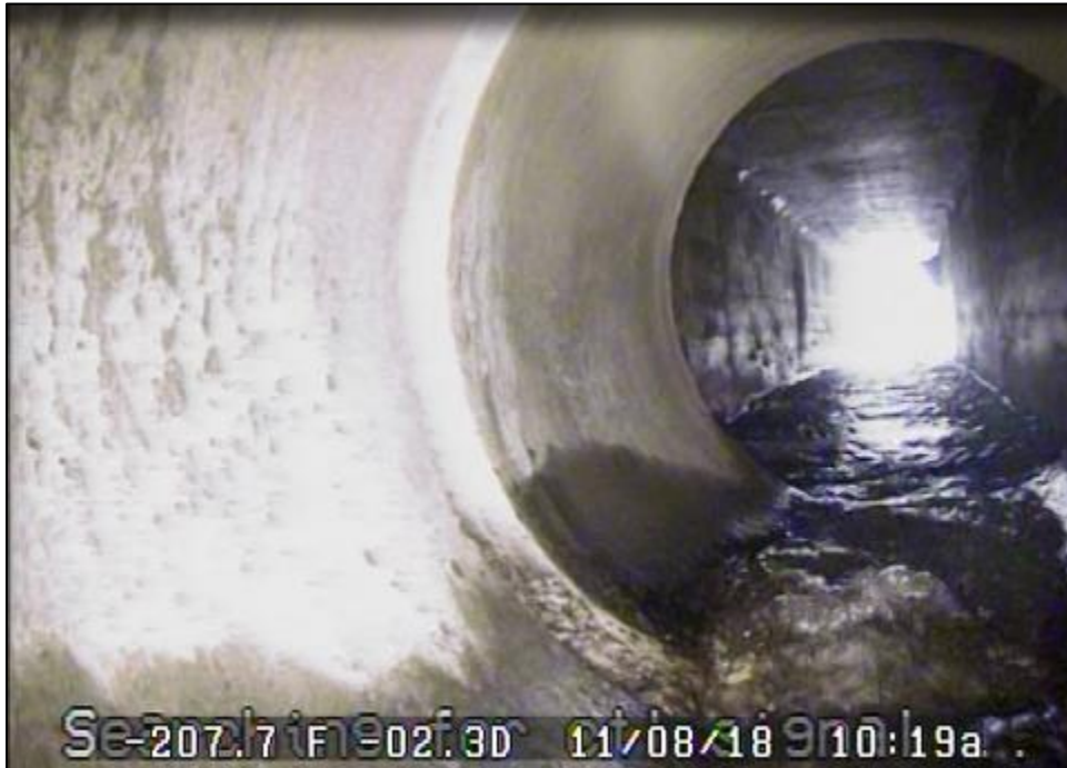
Discharge End of 36" RCP Into Box Culvert at Swanson Street
