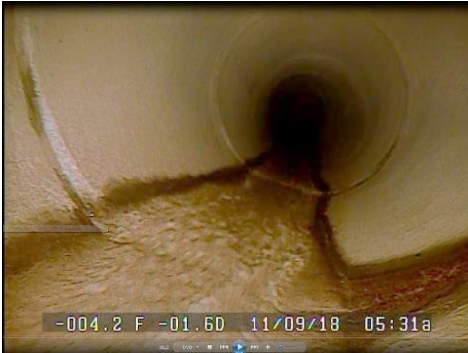
24" RCP Crossing Lafayette Street
