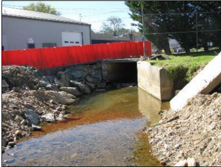
Outlet End of 6' x 3.7' Box Culvert
