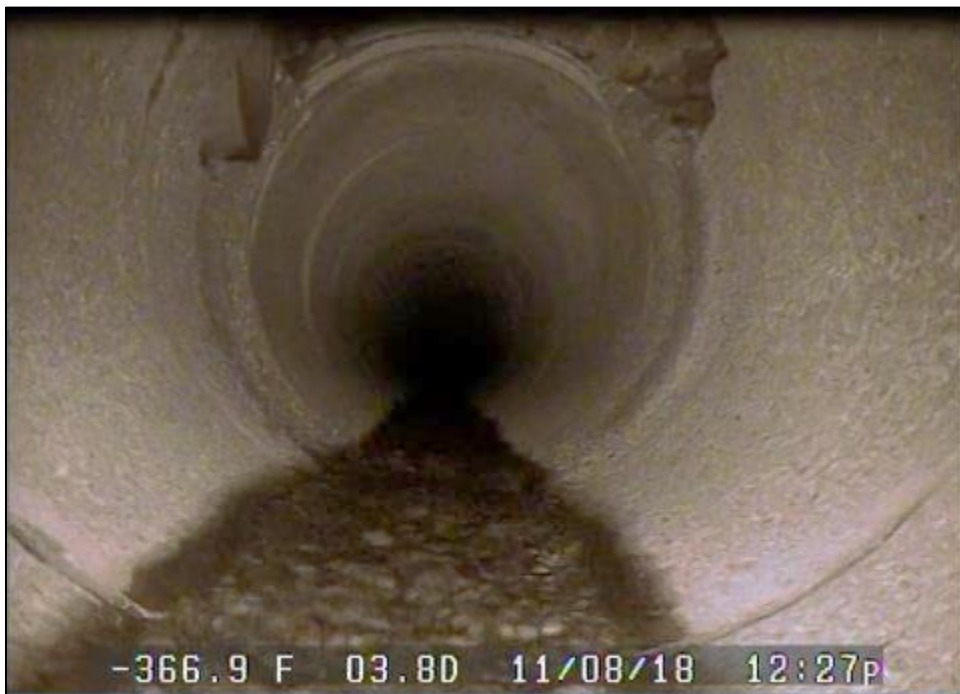
Storm Structure B2 in Carroll Street
