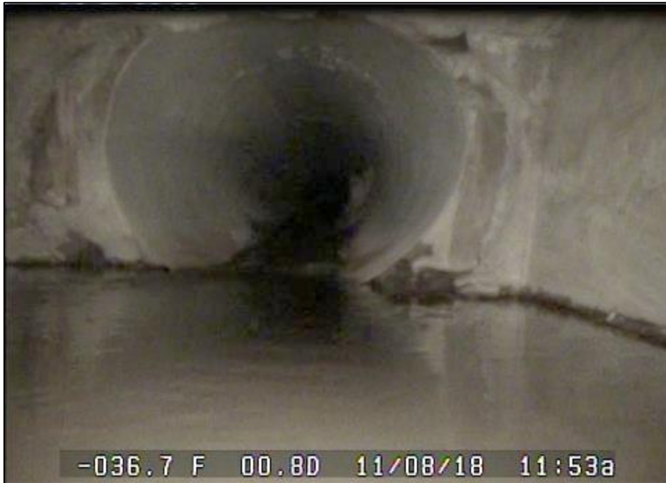
Transition from Box Culvert to 42" CMP at Depot Street
