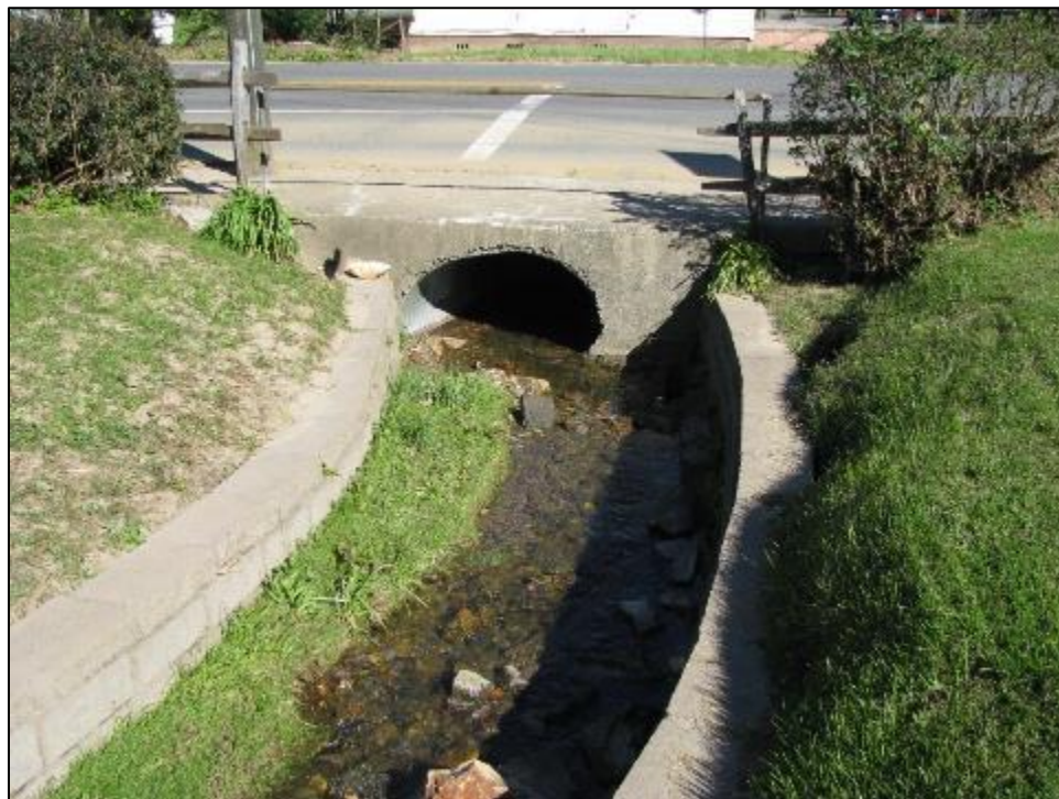
Inlet End of Arch CMP Near Swanson/McArthur Intersection
