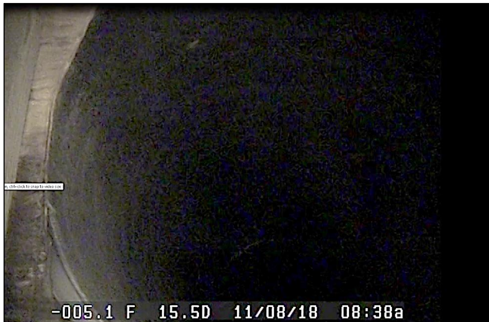
Inlet End of 60” HDPE Pipe at Galax Elementary Playground
