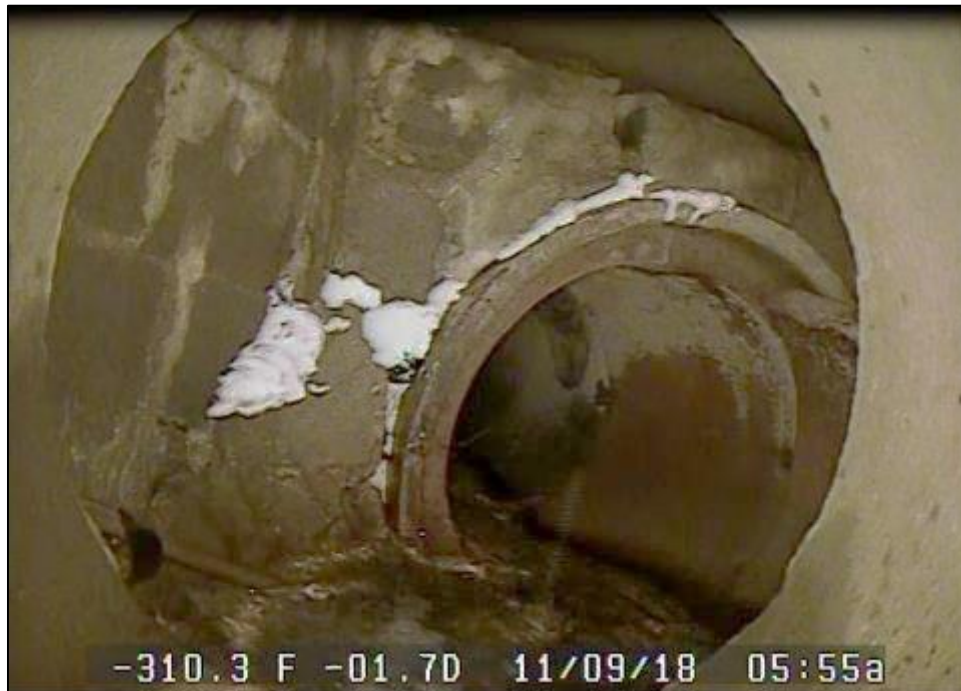
Transition from 24" RCP to 24" Terra Cotta in Alley
