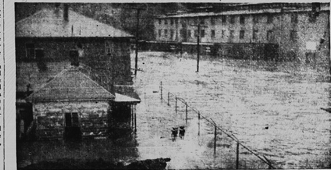
In the picture above is shown a view of the Vaughan Furniture Company factory here when the devastating flood of last Wednesday was at its height. The side of the factory shown faces the railroad and the street that passes the plant leading to the East-Stuart Drive intersection. Much damage was done to stocks of furniture in the plant by the inundation.—(Gazette Photo).
