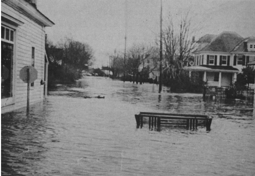
Flooding during the Ash Wednesday Storm of 1962. Photo printed in the Army Corp of Engineers Flood Plain Report for Wachapreague
