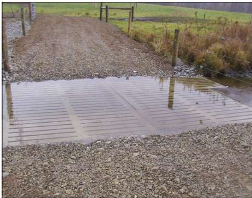
Hog panel stream crossing
