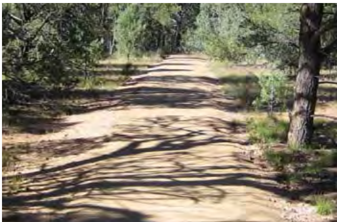
Resin-based stabilized material trail; Glorieta Pass Trail, New Mexico. Courtesy of Soil Stabilization Products Company, Inc.
