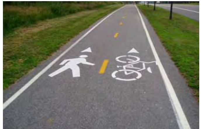
On-path pavement markings delineating pedestrian vs. bicycle routes. Courtesy of City of Roanoke
