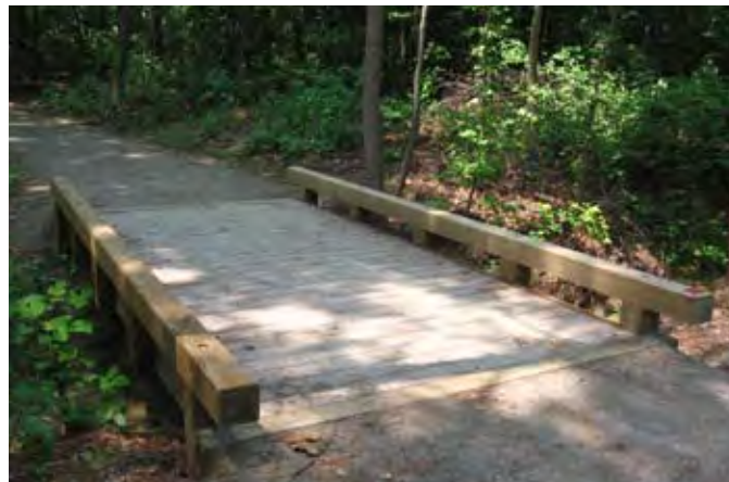
Boardwalk bridge on Government Center Trail in Chesterfield County, VA. Courtesy of DCR.
