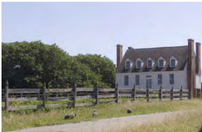
Trail to historic house at Chippokes Plantation. Courtesy of DCR.
