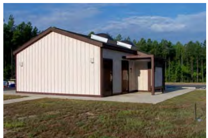
Large restroom facility. Courtesy of Virginia Horse Council.
