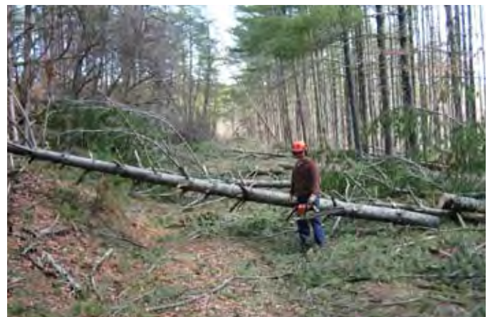
Clearing vegetation to widen a trail corridor. Courtesy of Roanoke Valley Greenways.
