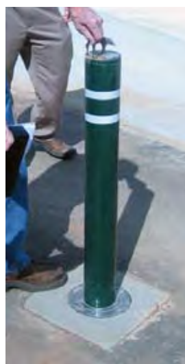
Left: Retractable metal bollards slide into a sleeve set in the ground when not in use. Courtesy of LPDA, Inc. Right: Removable bollards pull out of the ground completely. Courtesy of www.pedbikeimages.org /Dan Burden.
