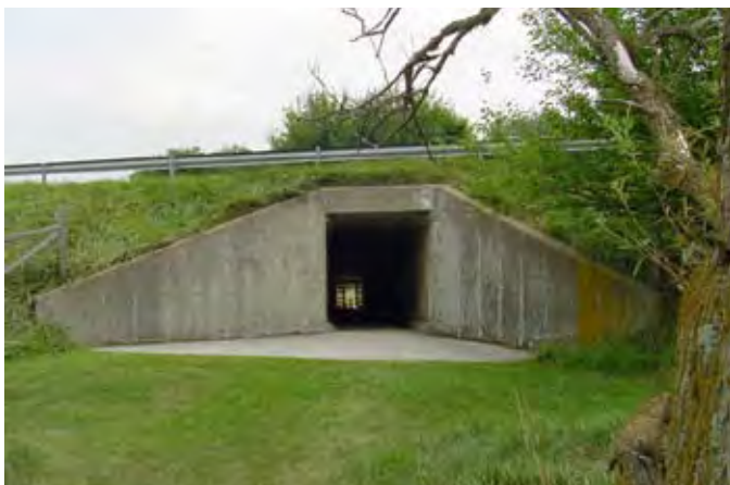
Tunnel on the New Market Trail. Courtesy of DCR.
