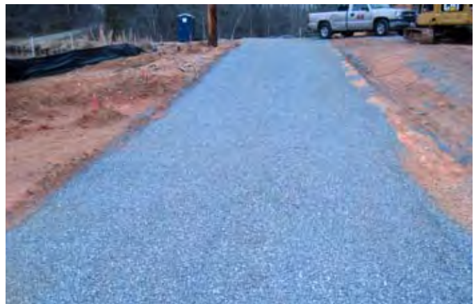
Chip and seal trail; Ivy Creek Park, Lynchburg, VA. Courtesy of LPDA, Inc.
