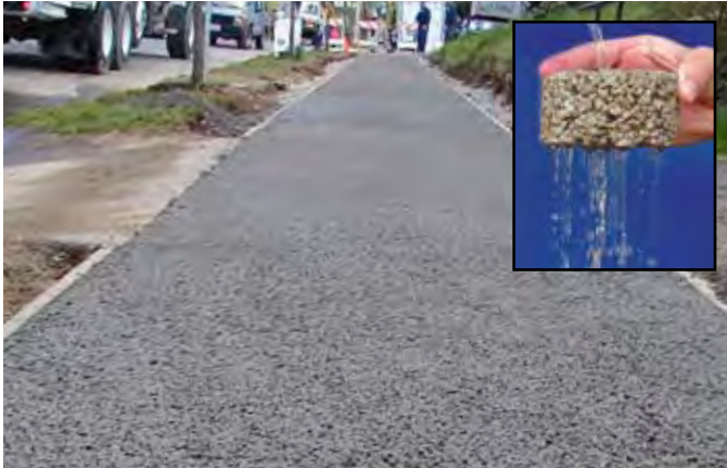
Pervious concrete sidewalk. Courtesy of National Ready-Mix Concrete Association at www.perviouspavement.org .
