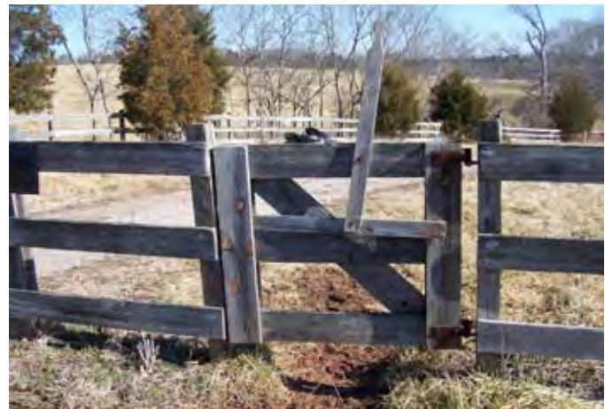
Gates with vertical handles allow equestrians to open and close the gate without dismounting. Courtesy of Virginia Horse Council.
