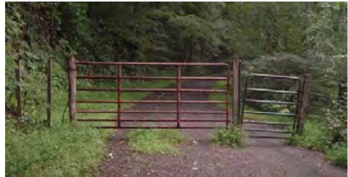
Double gate to allow independent use by both motorized and non-motorized trail users. Courtesy of AmericanTrails.org/Kentucky Rails to Trails Council.
