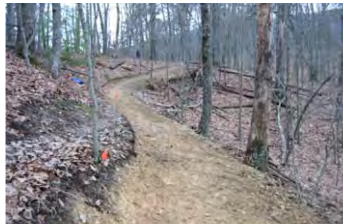
Hiking trail graded to shed water downslope. Courtesy of City of Roanoke.
