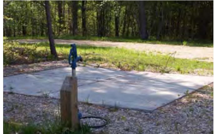
Simple concrete slab wash area with a yard hydrant. Courtesy of Virginia Horse Council.
