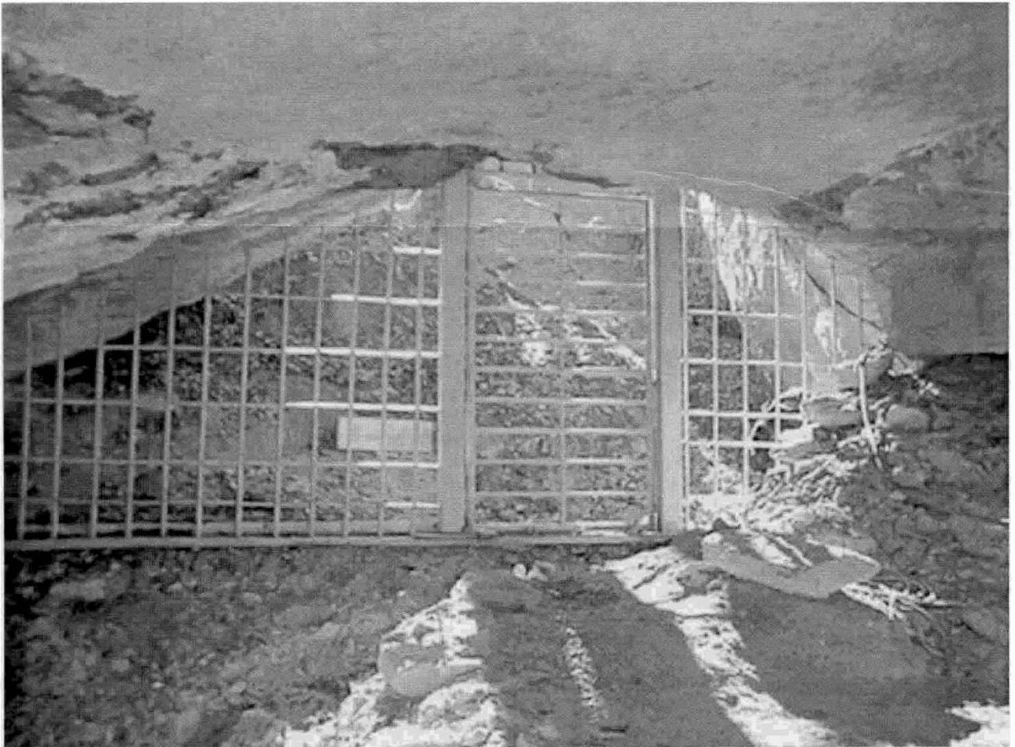
Figure 1: Entrance to Grays Cave, Russell County, Virginia. This gate was constructed by Danny and Laura McGlothlin. It is designed to thwart trespassers yet it allows easy access for bats that inhabit the cave.
