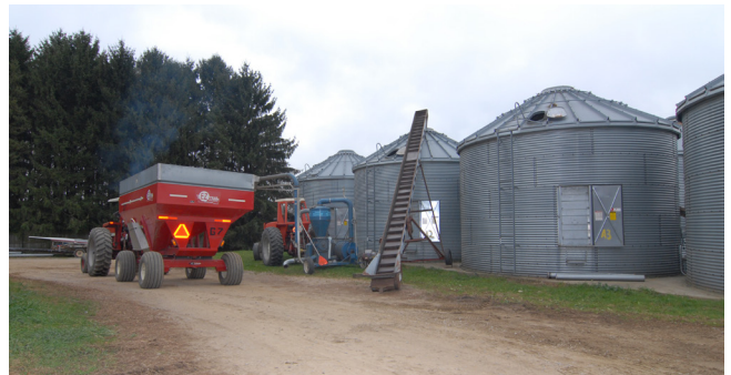
Figure 5. Exterior of Seed Drying Bins
