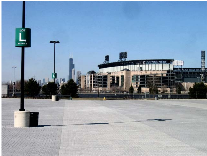
Pave block parking with reservoir storage beneath (at U.S. Cellular Field in Chicago)
