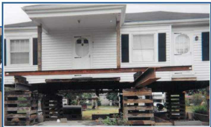
Photo II-2: Town of Glasgow, Flood Mitigation Project, 1997-2002
