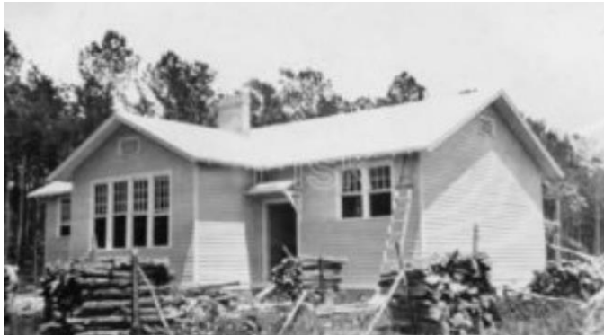
FIGURE 6: FRONT OF THE ANTIOCH ROSENWALD SCHOOL DURING CONSTRUCTION IN 1927.
