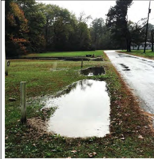
Southward facing view along Antioch Road taken from in front of the Antioch Rosenwald School. The photograph was taken recently following a nominal rain event with less than 0.5" precipitation and is representative of the regular conditions at the site. The level of ponding in the roadside ditches and the yard in front of the school building are a constant challenge for daily operations at the site.
