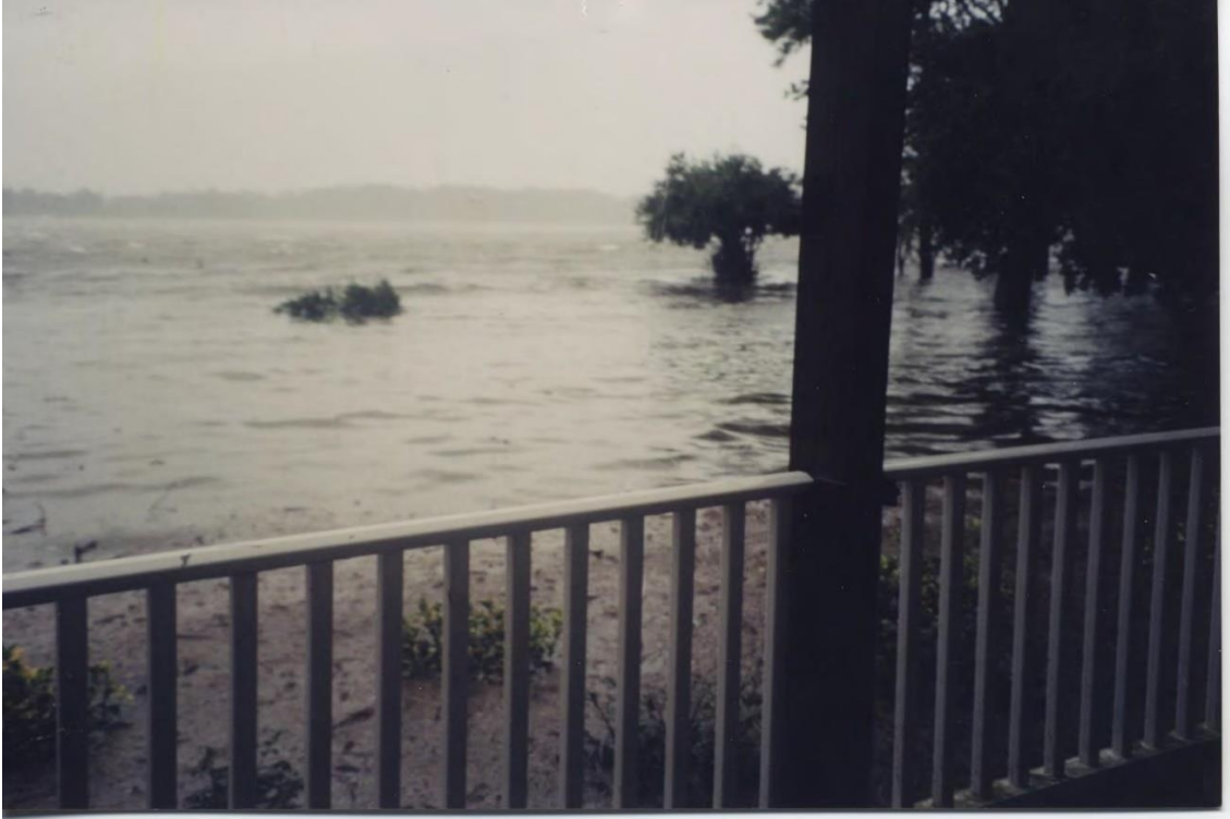
The below photos show the damage from Hurricane Isabel in 2003. The water reaches the house during the hurricane.
