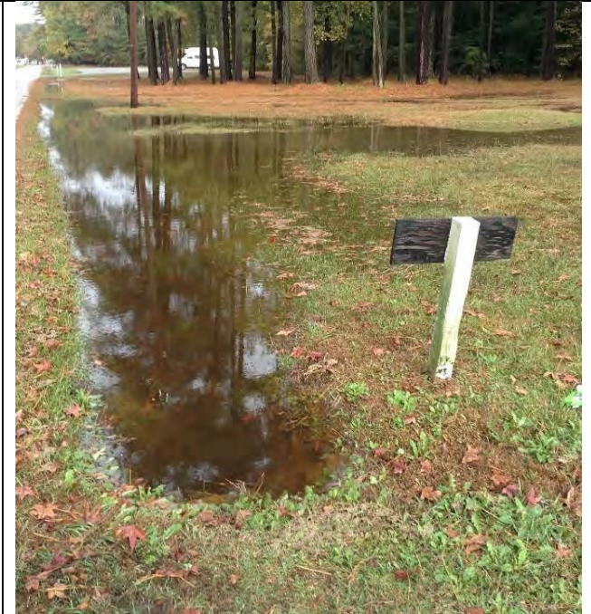
Northward facing view along Antioch Road taken from in front of the Antioch Rosenwald School. The photograph was taken recently following a nominal rain event with less than 0.5" precipitation and is representative of the regular conditions at the site. The level of ponding in the roadside ditches and the yard in front of the school building are a constant challenge for daily operations at the site.
