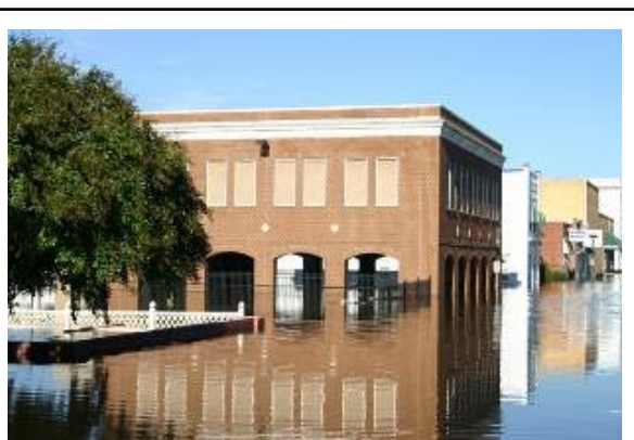
Downtown Franklin during the October, 2006 flood. Source: City of Franklin photo
