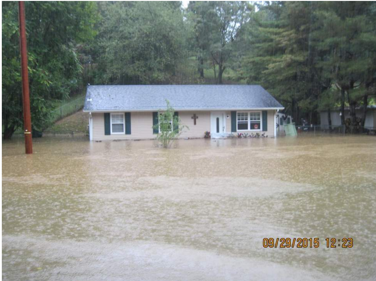
Figure 1 - Flooding of residence along Phlegar Street
