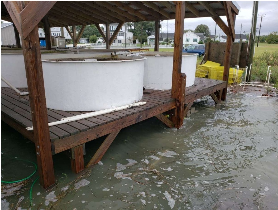
Photo 2: Flooding of TNC's Marine Habitat Restoration facility during an average storm event in spring 2021.
