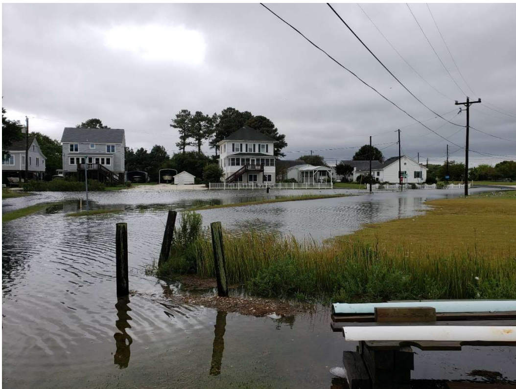
Photo 3: Flooding of Sunnyside Road and Broadwater Circle.
