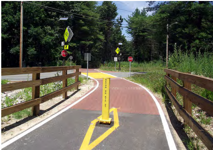
What is wrong with this photo? Don't use yellow to mark the crosswalk through the roadway. Continuing the brick surface with white striping would work.
