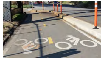
What is wrong with this photo? All crosswalks must be bordered with retroreflective white striping. Signs do not conform to MUTCD guidelines.
