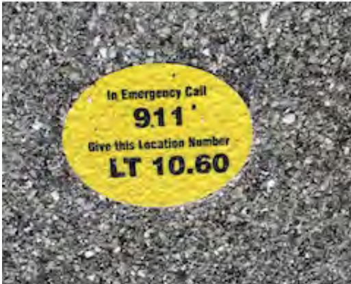
Mile markers on pavement. LT 10.60 represents the Legacy Trail 10.6 miles north of the Venice Train Depot in Sarasota, Florida.
