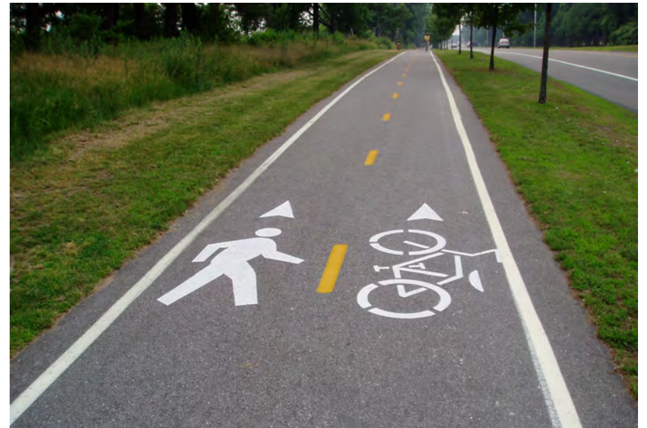
What is wrong with this picture? As a rule of thumb, slower traffic keeps to the right. Pavement markings can be a maintenance issue, particularly if your shared-use path is plowed in winter. Consider whether edge and center lane striping are really needed.
