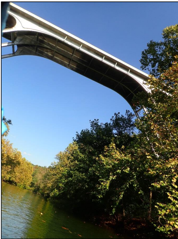
Image 26. Interstate 64 above the Maury River.
