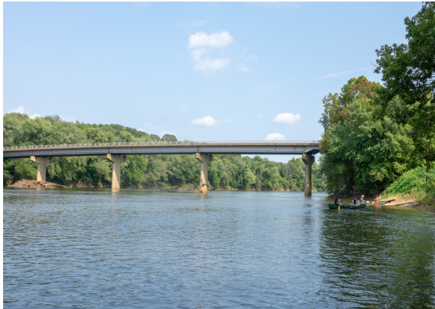
Figure 16: Columbia Road Bridge
