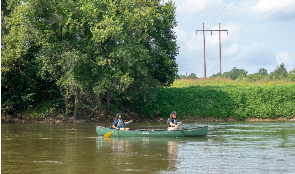
Figure 15: Electrical transmission lines near Columbia, Va.
