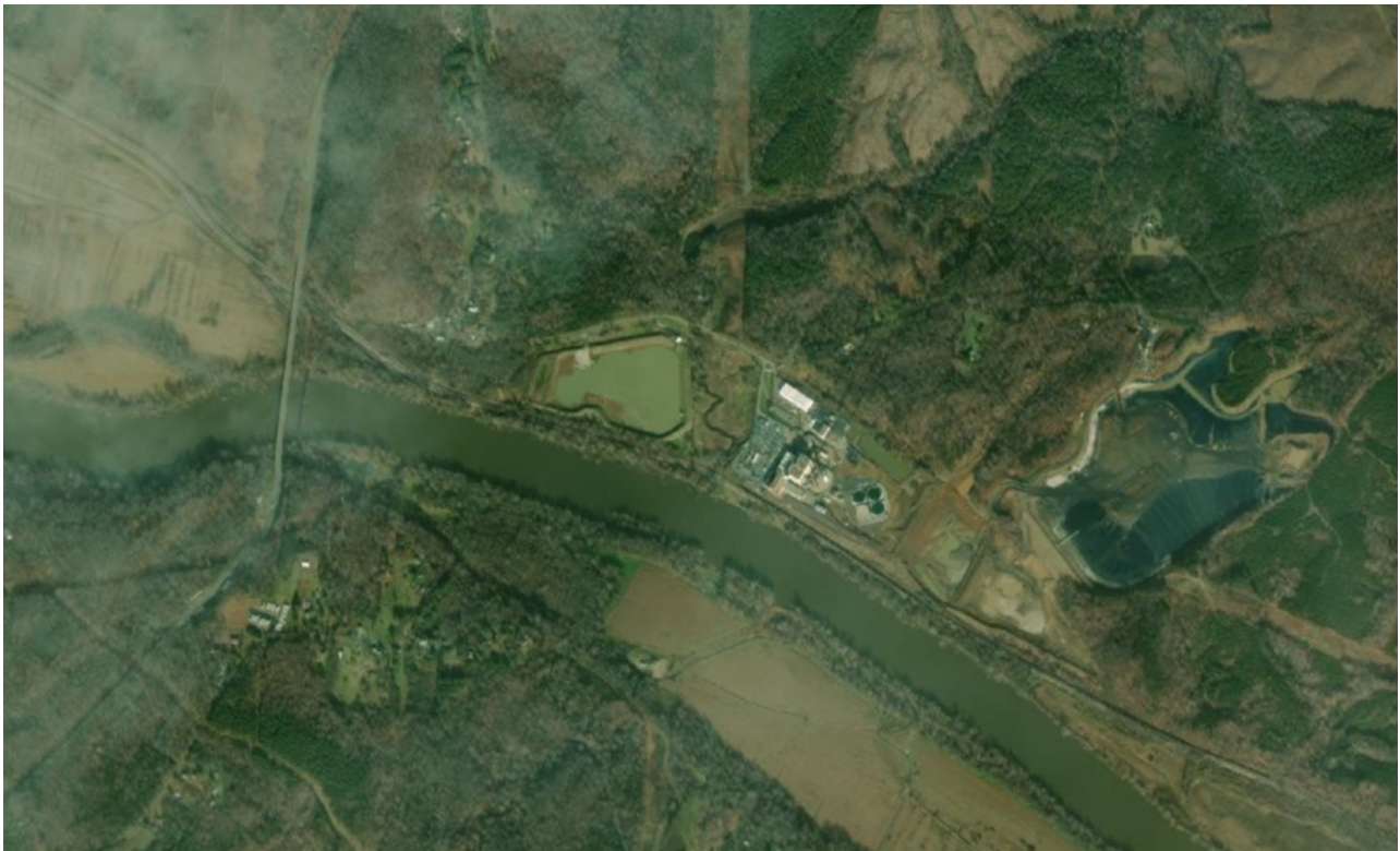
Figure 8: This map shows Bremono Bluff Powerplant which is located just after the boat ram that in New Canton, Va.
