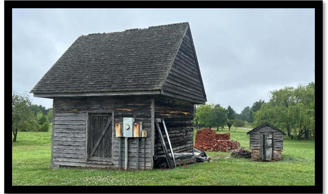
Extant smokehouse and wellhouse
