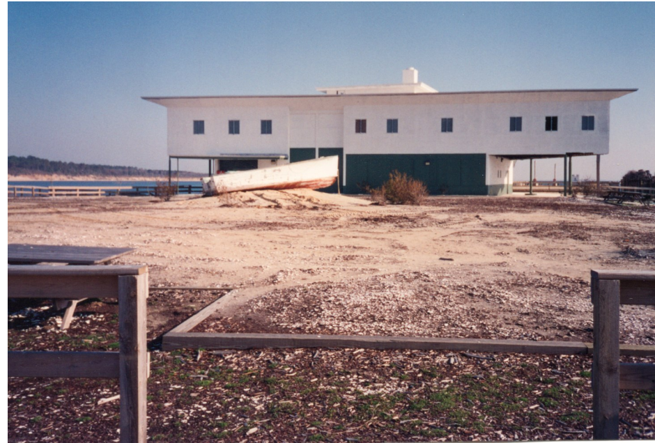
Left: the terminal building soon after the park opened in 1992—originally the park planned to use this as a visitors center, but structural and asbestos issues mandated its demolition
