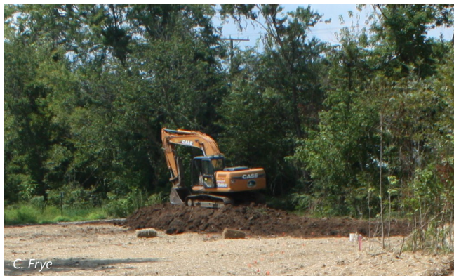
Figure 4-1: Amendments being incorporated into the surface soils on a re-vegetation project.
