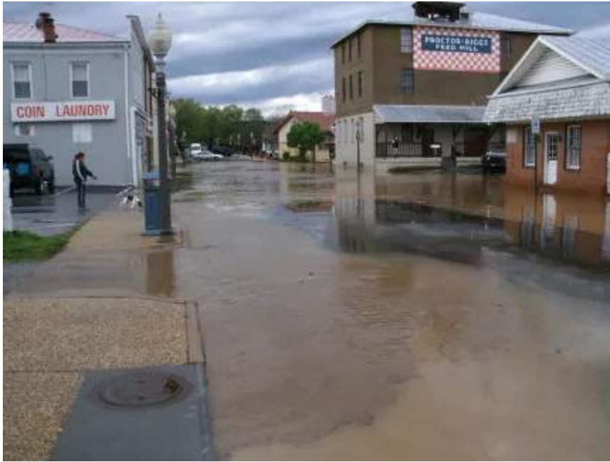
Main Street/Downtown – Flooding from Happy Creek
