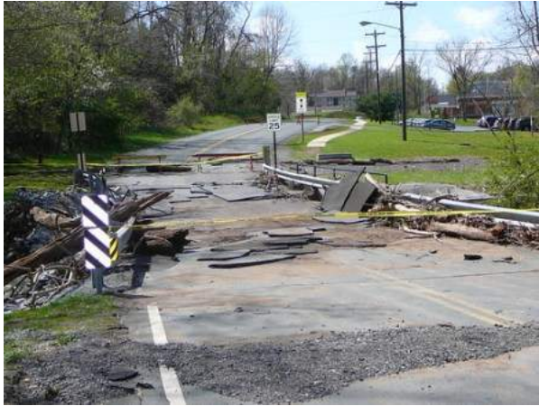
Criser Road Bridge over Happy Creek
