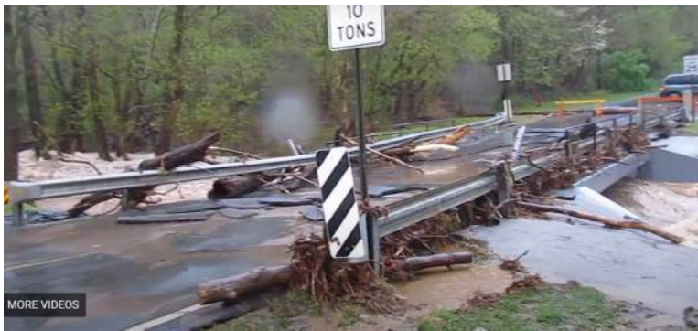
Criser Road Bridge over Happy Creek
