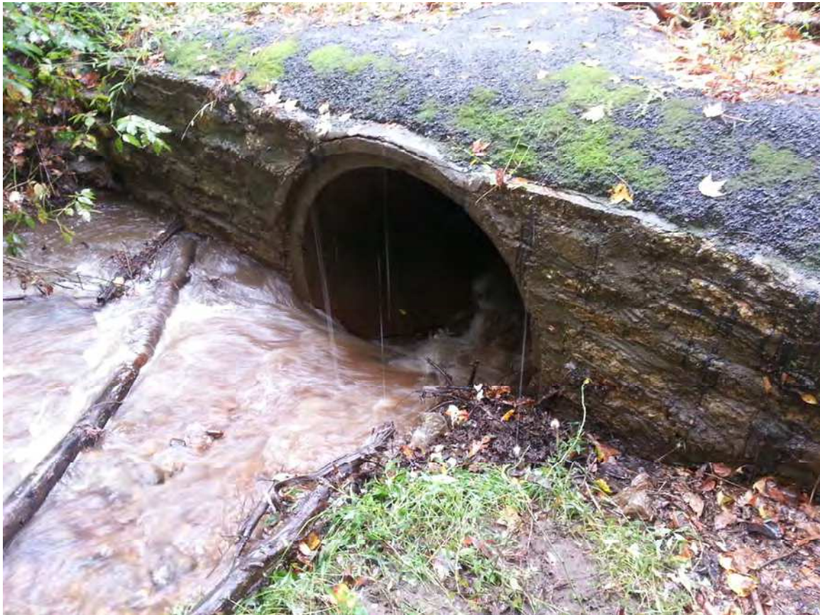
Cherokee Avenue crossing inlet.
