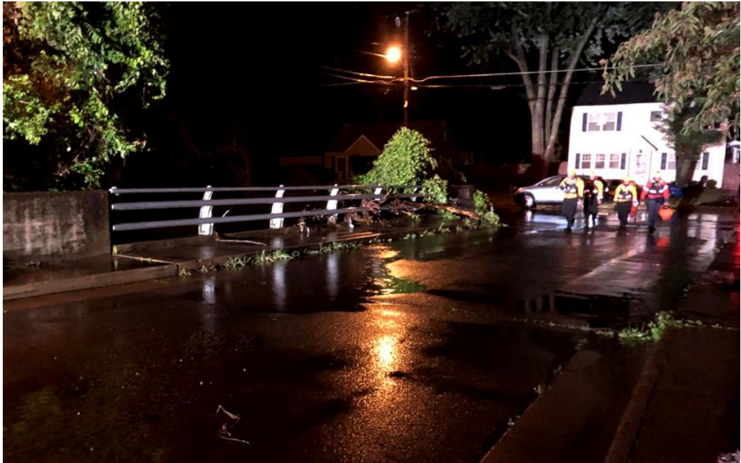
Photo 4: July 2020 Storm Event, Tripps Run at Holloway Rd
