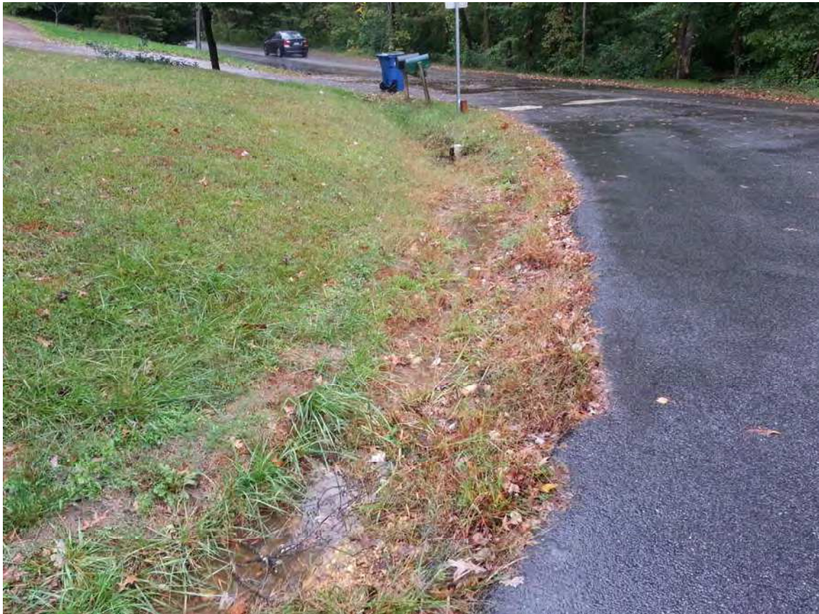
Ditch upstream of 8th Street and Chowan Avenue.
