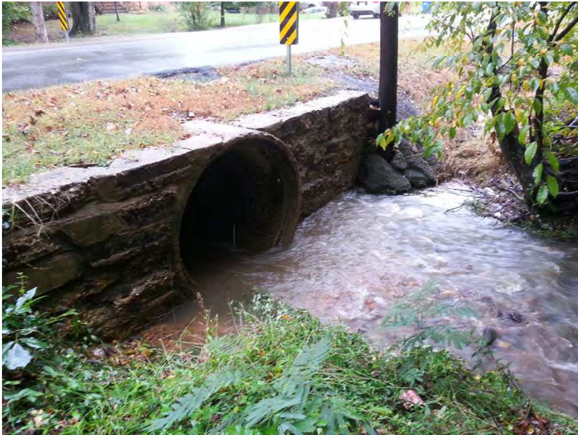
Chowan Avenue crossing inlet.
