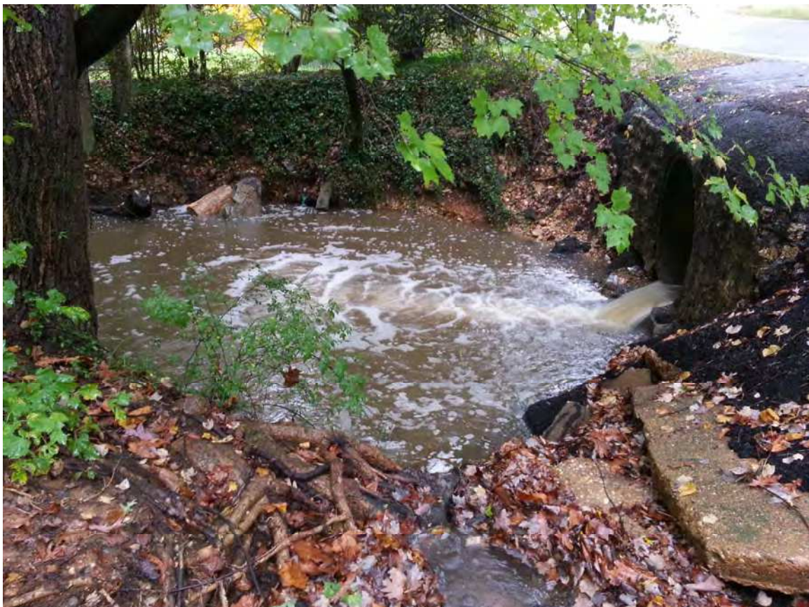
Cherokee Avenue crossing outlet.
