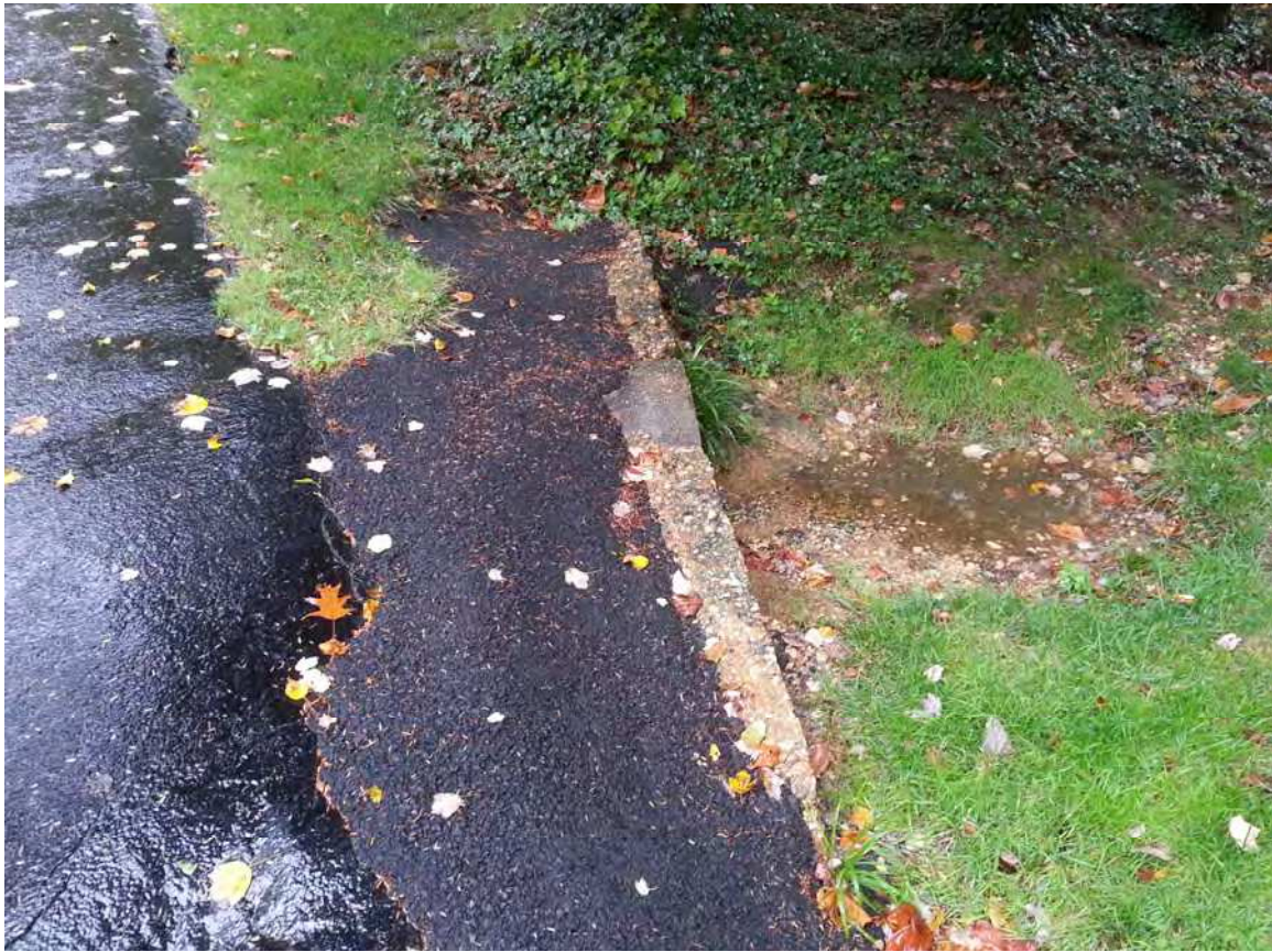
Drive way culvert
