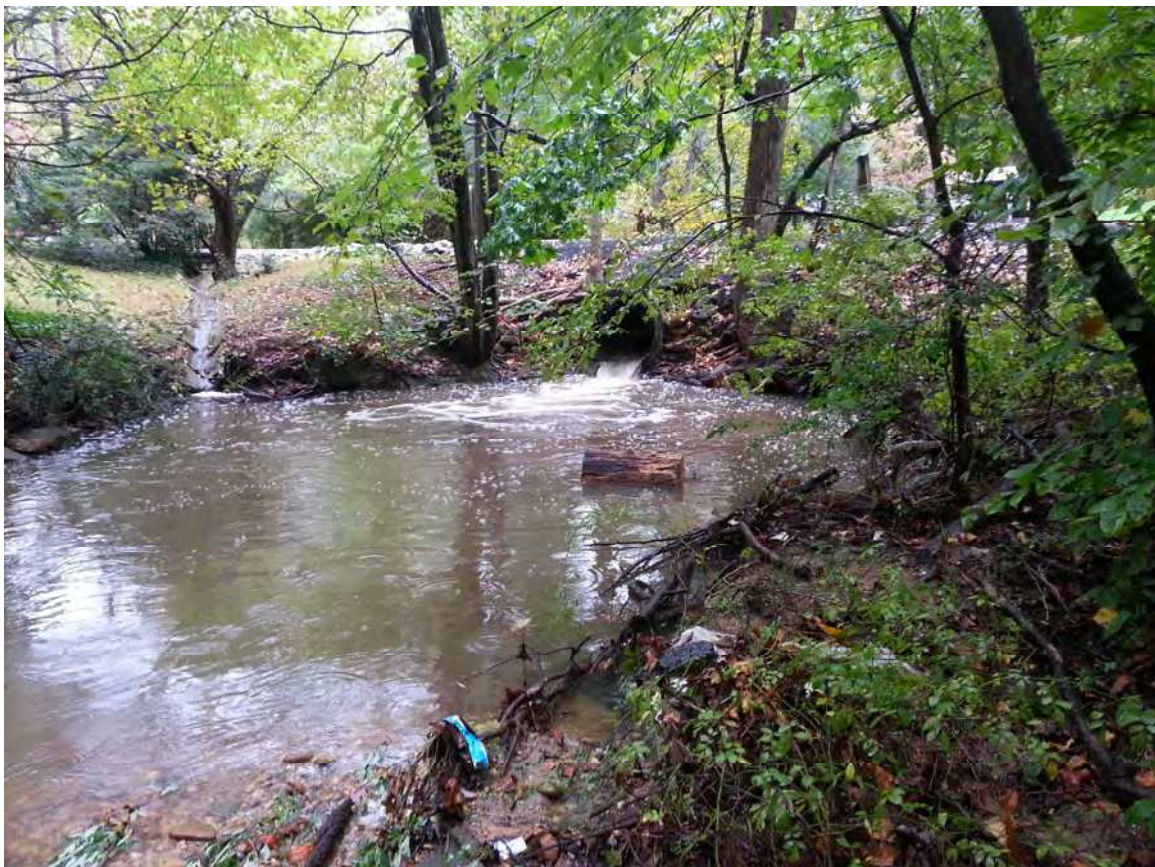
8th Street crossing outlet.
