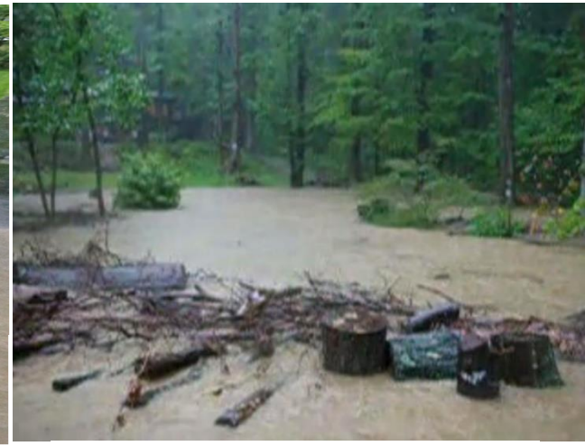
Overtopping at Chowan Avenue (September 08, 2011) (image from VDOT)
