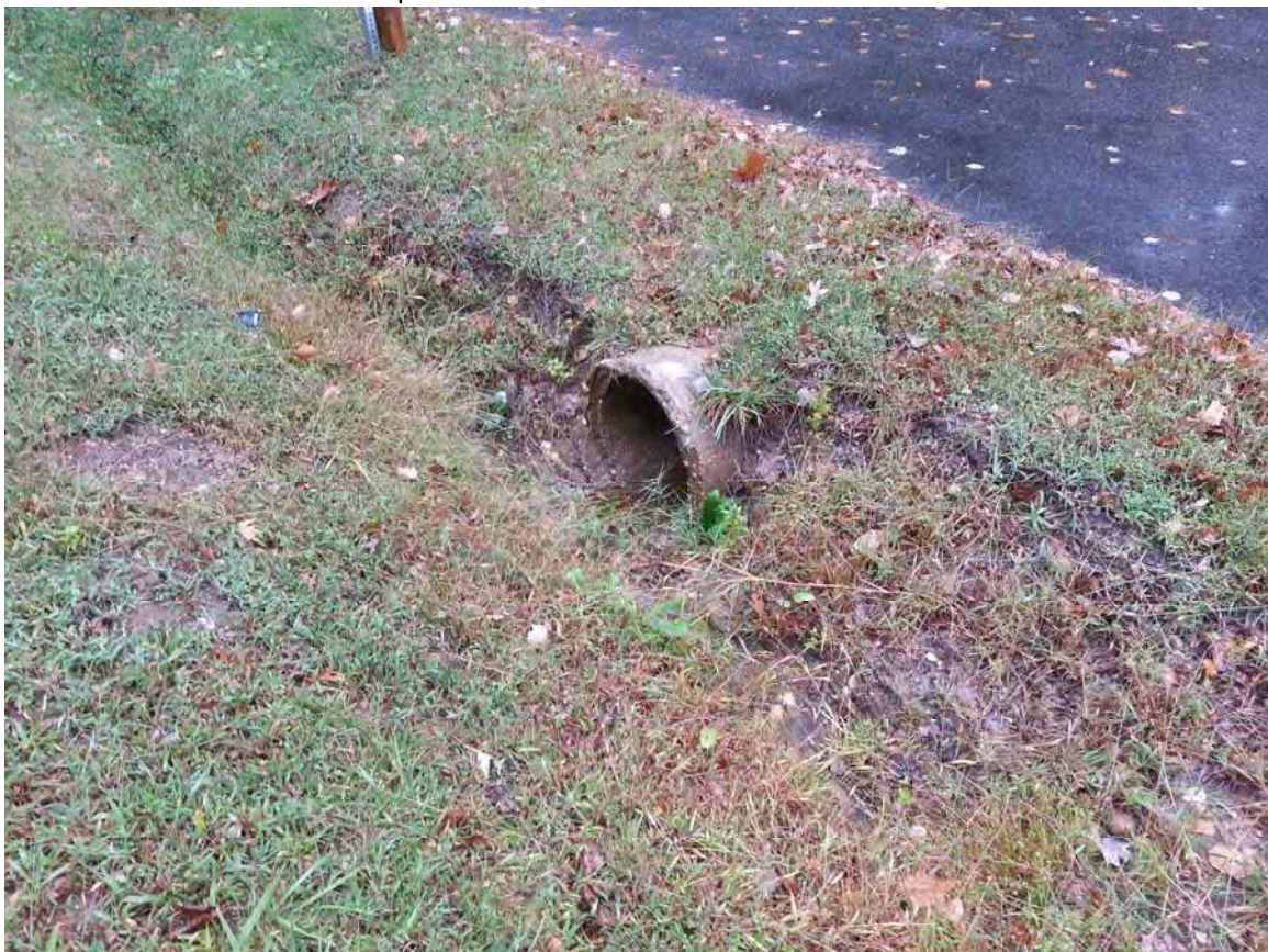
8th Street and Chowan Avenue crossing inlet.
