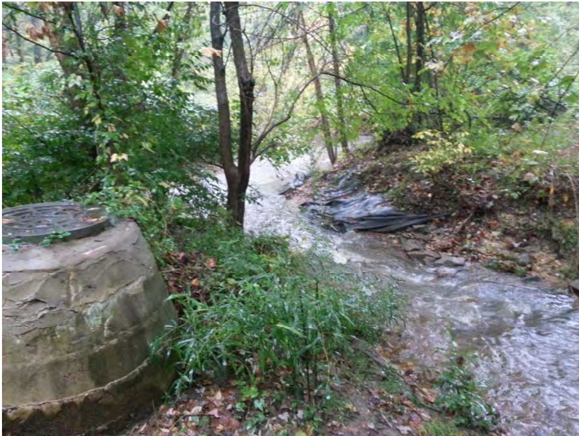
Junction of Tributary and Turkeycock Run
