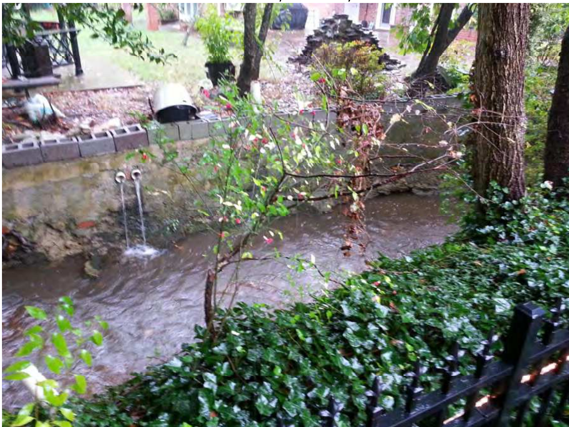
Access to channel from private property
