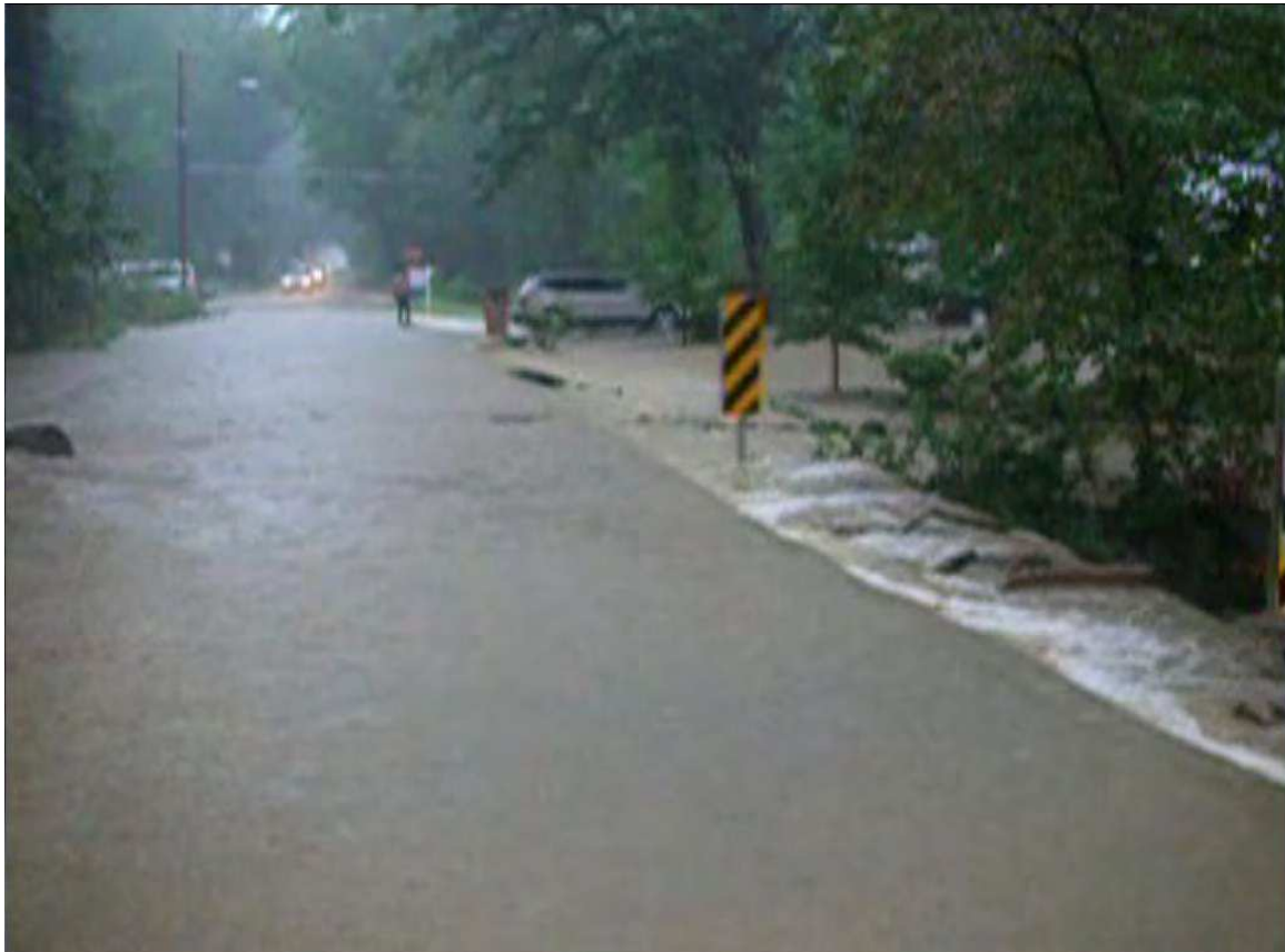
Overtopping at Chowan Avenue, impacting private properties (taken 2011-09-08)
