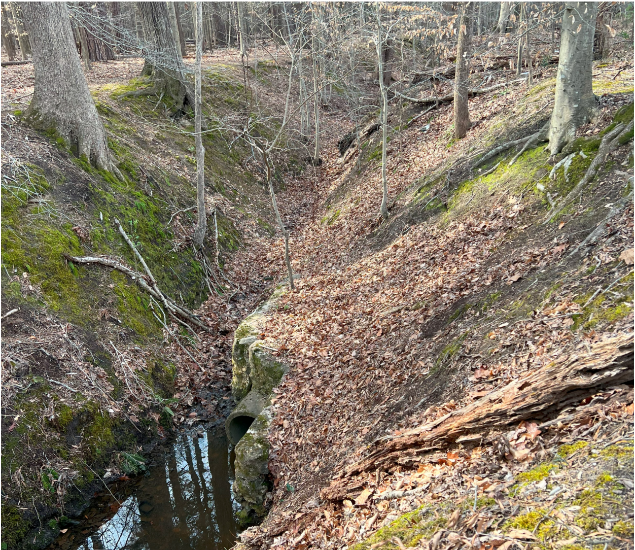
Figure 3. S. Whitehill Drive Storm Sewer System Outfall.
