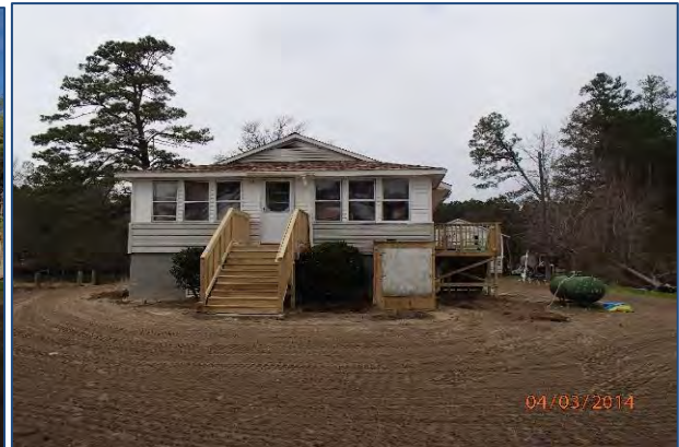
Figure 78: House in Hayes, Gloucester County - AFTER elevation.
