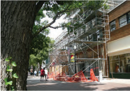
Mixed-Use redevelopment underway downtown.
