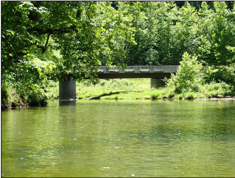
Image 26. Bridge crossing the Pound River. The bridge is Lower Georges Fork Holw.
