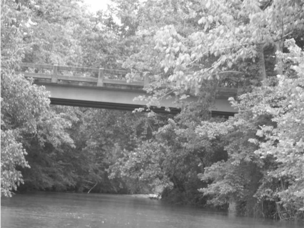
Figure 7 Route 695 bridge crossing the South Mayo River
