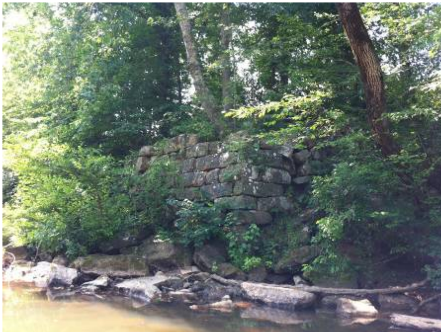
Image 15: Original stone abutments of Anderson's Bridge at Riceville "canoe landing"
