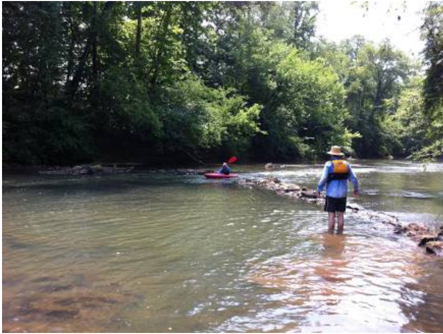
Image 14: Wing Dams at Cow Ford Bridge.
