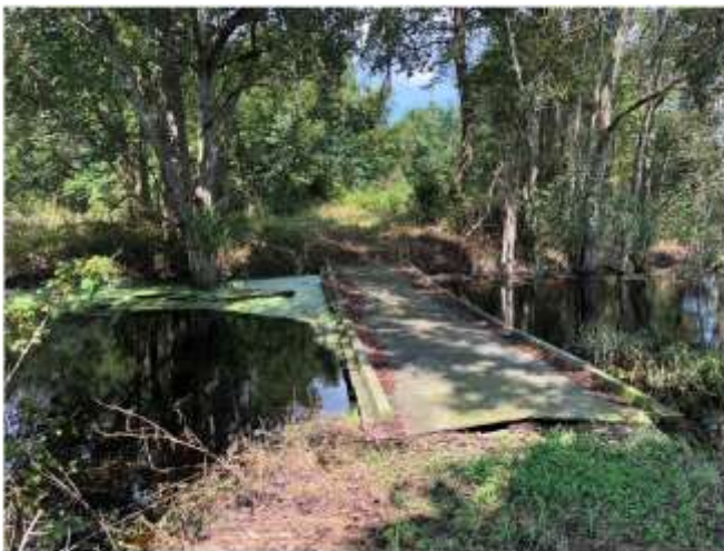
Bridge over canal to access hardwood forest area
