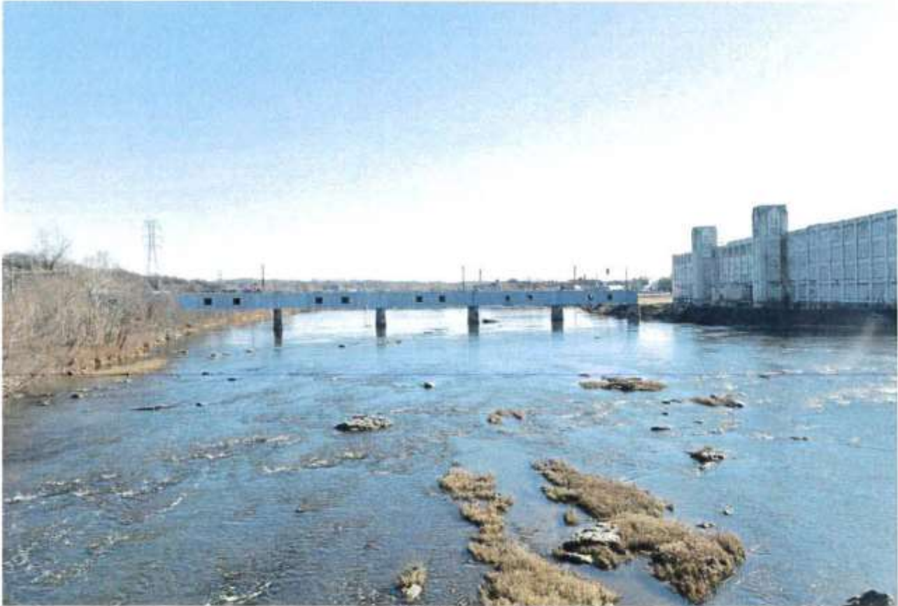
Covered Pedestrian Bridge Photo Credit: Register and Bee
