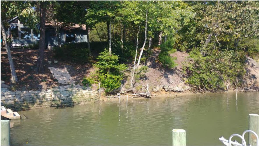
Shoreline. Envirolok Bags are shown on the right and on the left is the eroding shoreline where the Envirolok Bags are planned to be installed to the property line.
