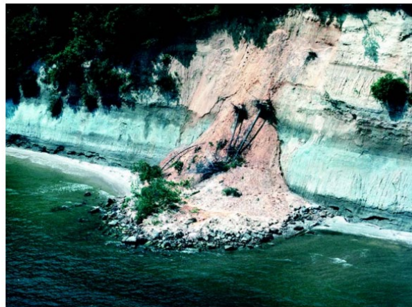
Figure 6-11: Nomini Cliffs Landslide
