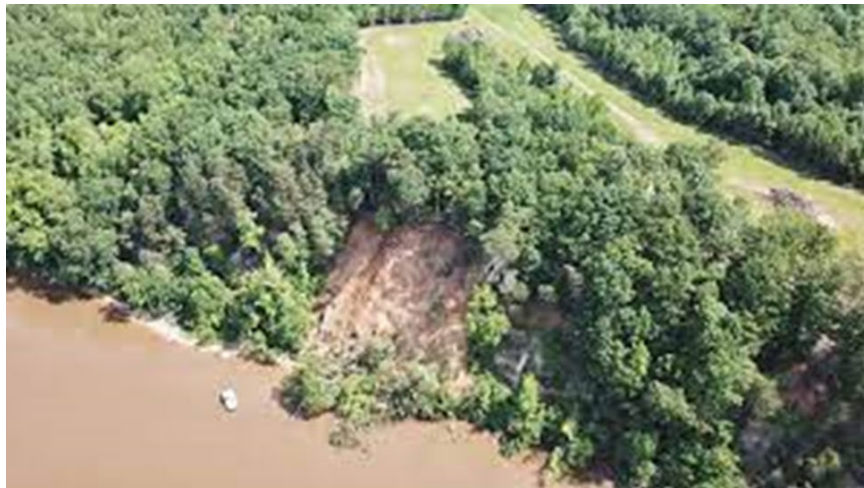
Figure 6-12: Fones Cliffs Landslide May 24, 2018
