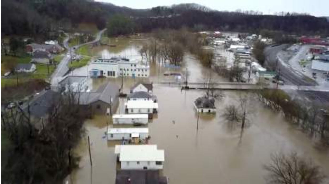
Figure 626: Flooding in Richlands, February 2020
