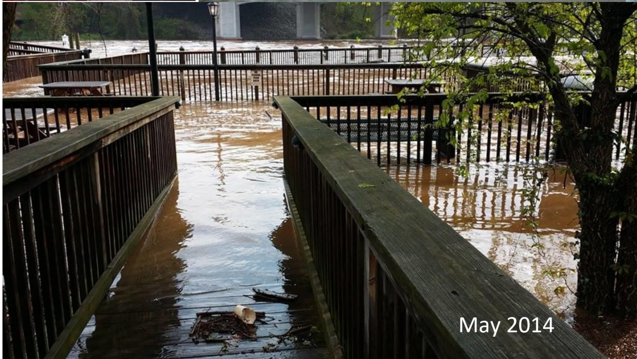
Recent Flooding events in Occoquan
