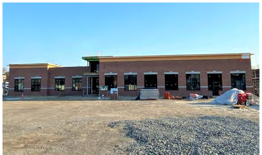
Construction of the Eastern Shore of Virginia Regional Library
