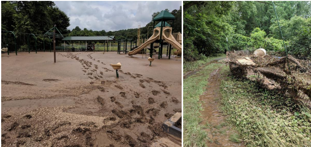
Azalea Park Flood Damage, May 2018
